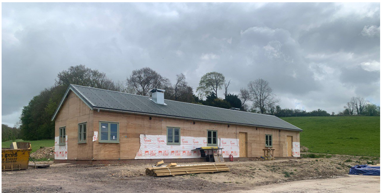
Figure 3: The barn under construction (in accordance with Class Q consent)
