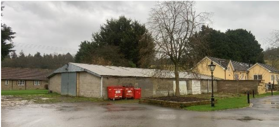
Photograph of the 'Tractor Shed'
