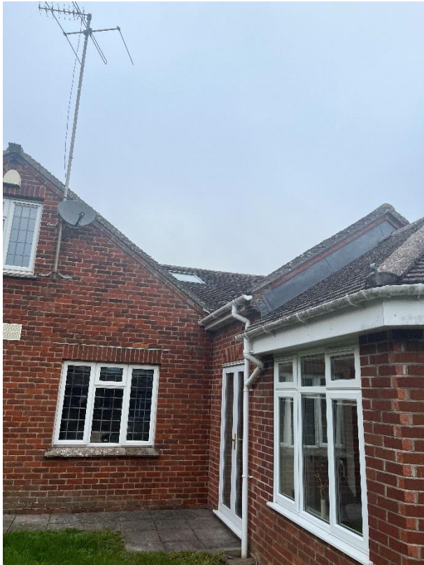
Existing south elevation of property with varying rooflines - location of 1 no proposed dormer
