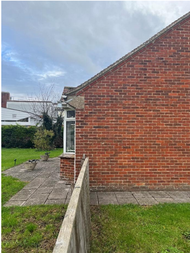
Side-on view of west elevation of existing property with Telephone Exchange in background
