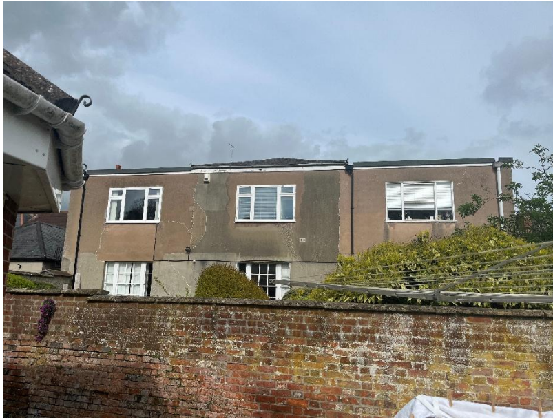
Flat roof two storey elevation of significant scale and massing to adjacent property east of site (3)
