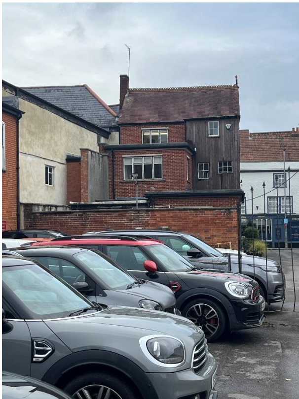
Flat rooves at varying elevations on modern extensions to rear of listed buildings north east of site (1)
