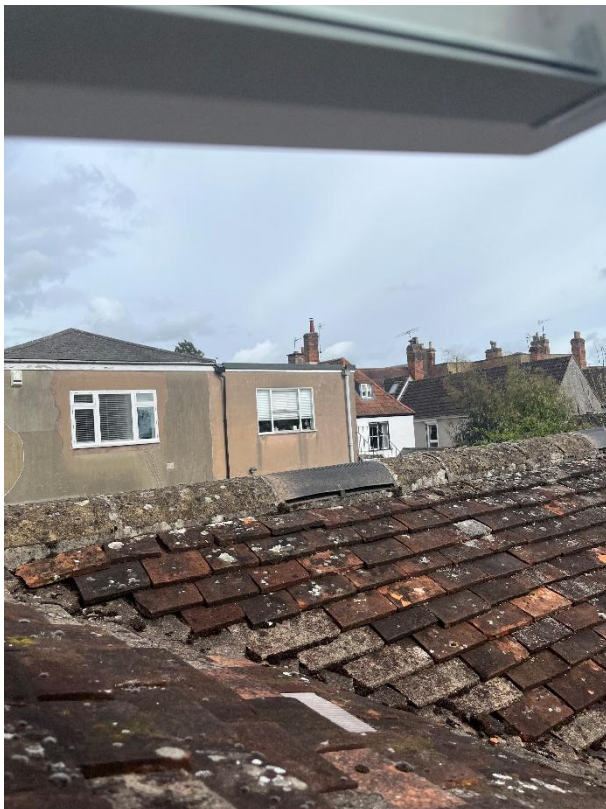
Flat roof two storey elevation of significant scale and massing to adjacent property east of site (2)
