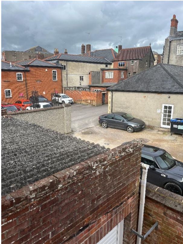
Flat rooves at varying elevations on modern extensions to rear of listed buildings north east of site (2)
