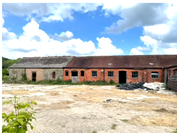
Figure 4. South-east elevation of Barn 1
