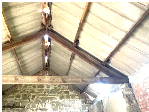
Figure 14. Big hole in roof
