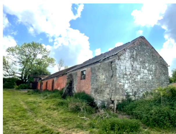
Figure 7. SW and NW elevations of Barn 1
