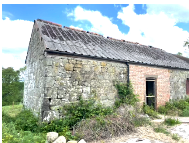
Figure 6. Close-up of SE & SW end elevations
