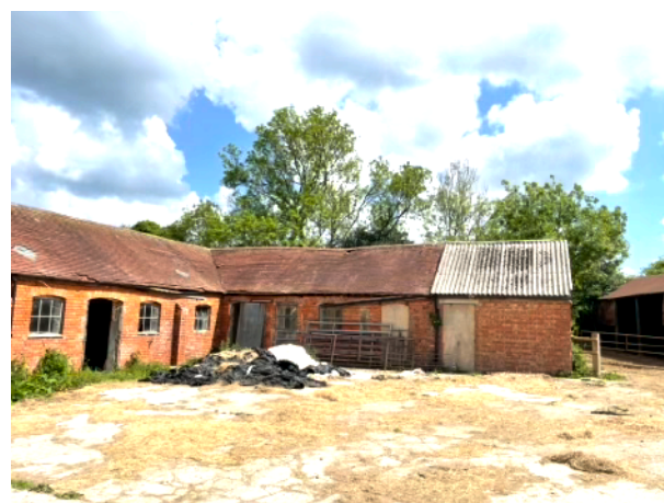
Figure 5. SE & SW elevation of Barn 1
