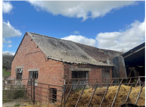
Figure 9. View of Barn 2 - SW & SE
