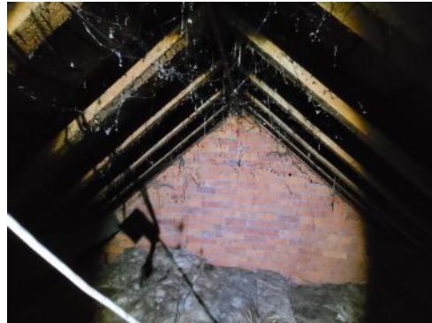
Photo 6: An internal view of the loft void.
