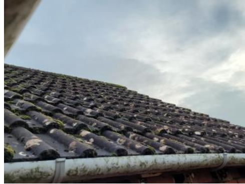
Photo 2: Well fitted concrete interlocking tiles.
