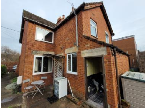
Photo 1: View of the building from the south-west.
