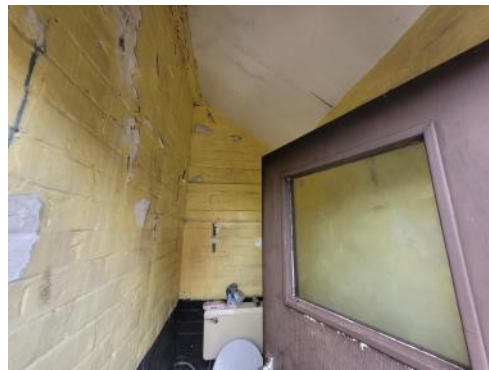
Photo 10: An internal view of the WC building showing boarded ceiling.
