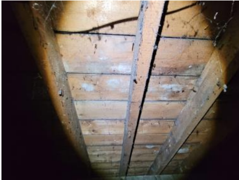
Photo 7: Wooden boarding beneath tiles.
