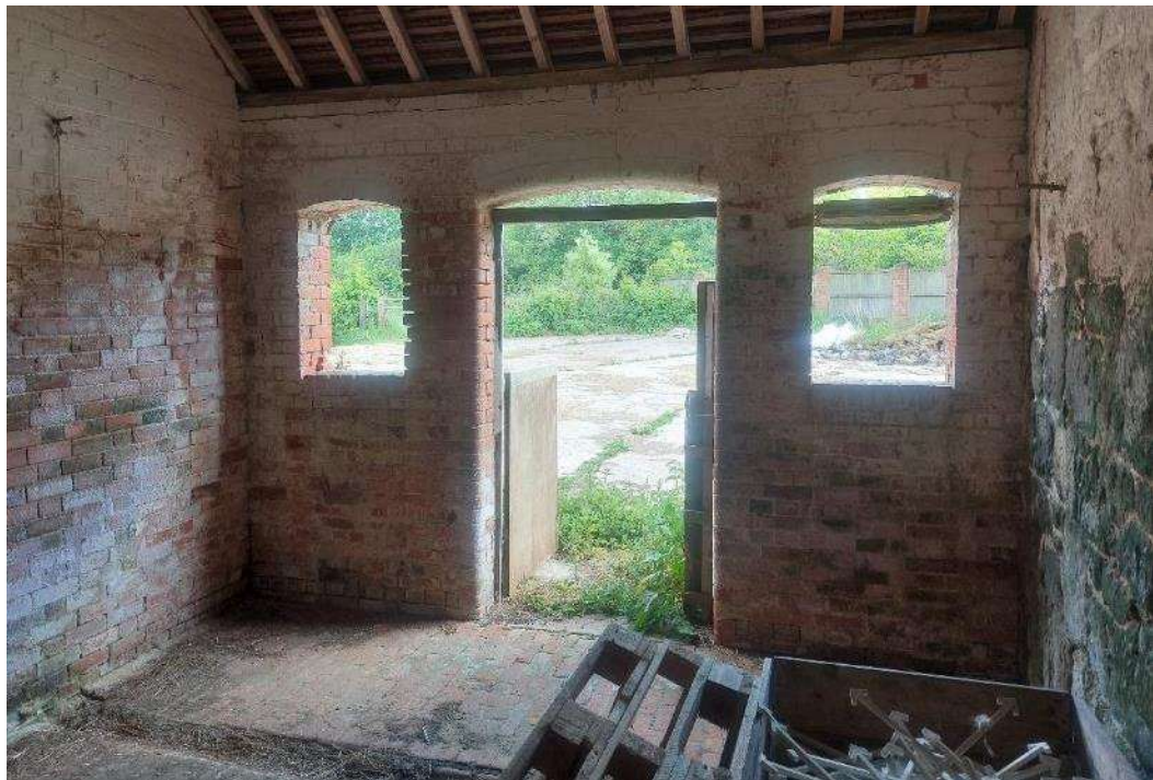
Figure 12 Interior of the stable adjacent to the barn, looking towards the front wall.
