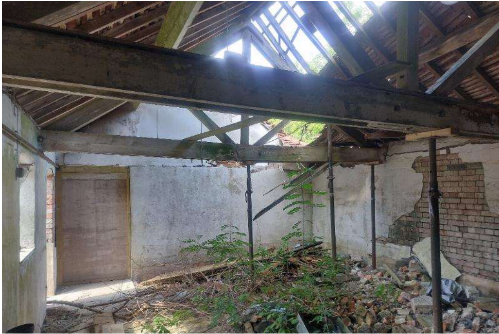
Figure 15 The interior of the east range looking north.
