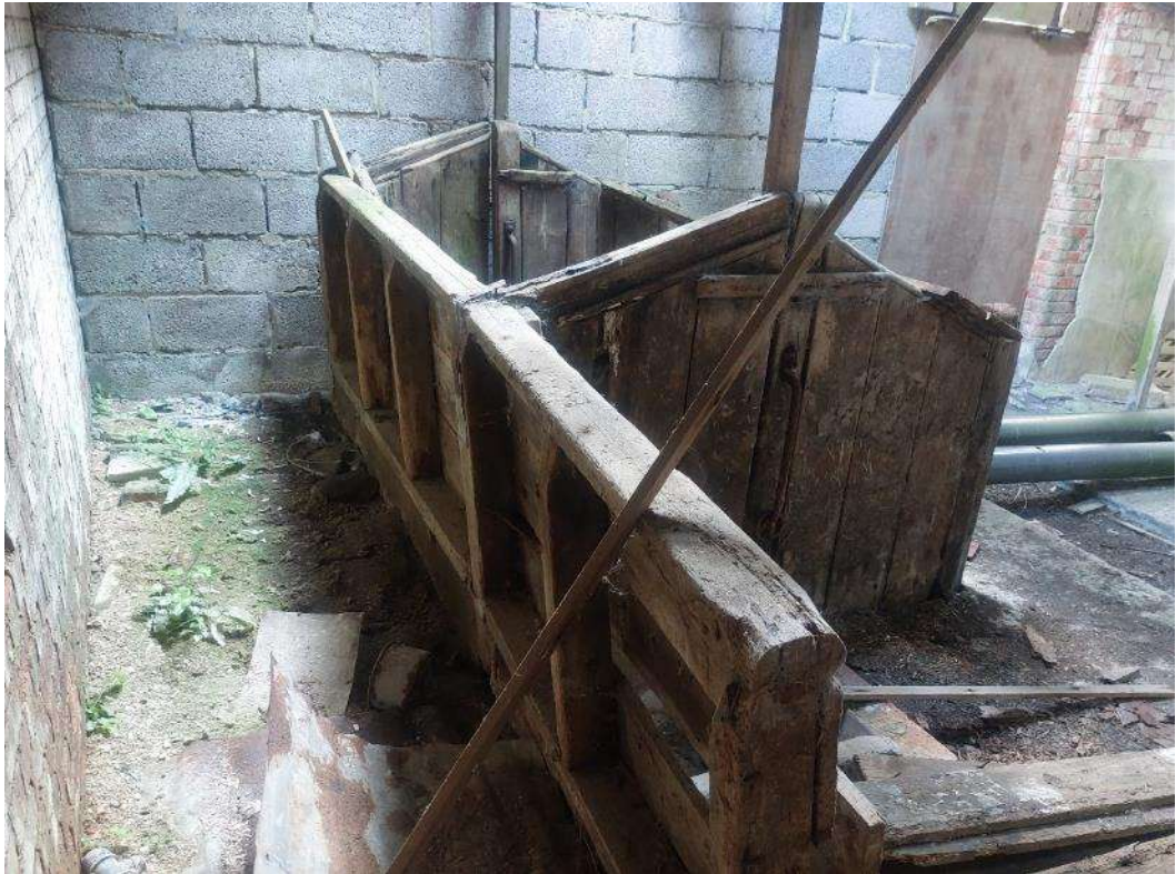
Figure 14 A section of surviving timber stalls with the feeding passage along the inside of the outer wall.
