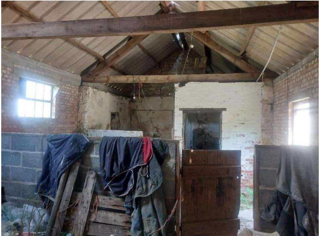
Figure 8 Barn interior facing east.
