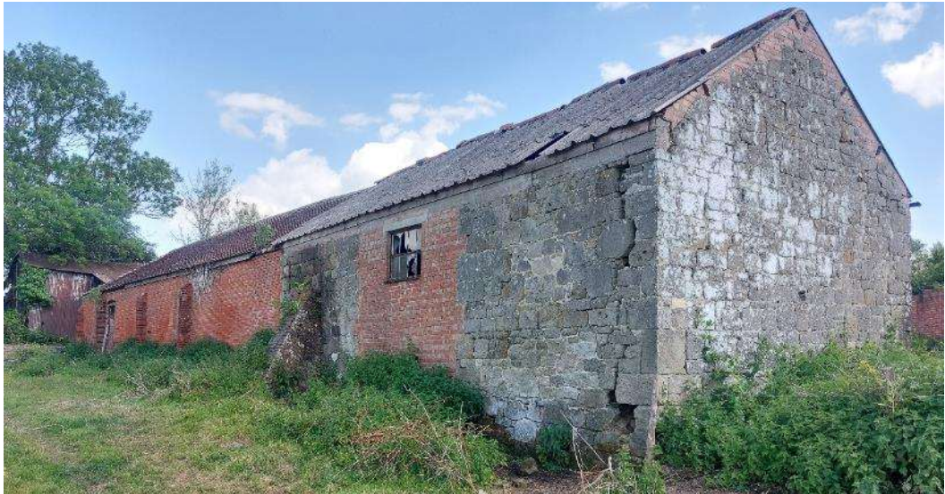
Figure 7 Barn, north and west elevations.
