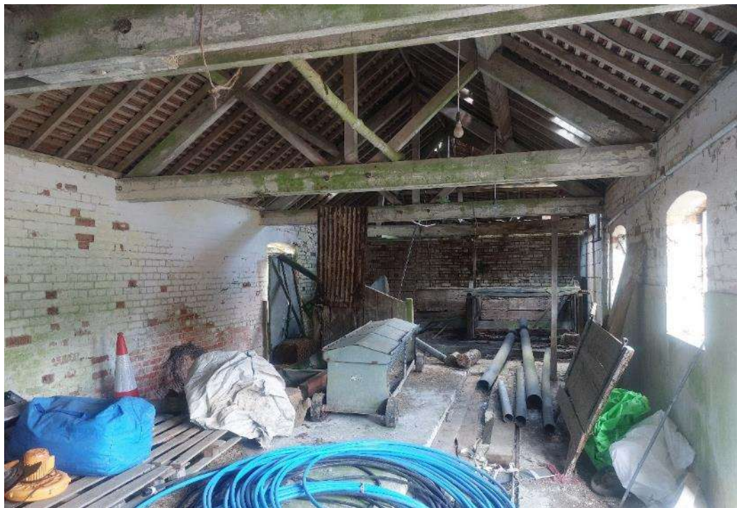
Figure 13 The interior of the cow shed within the main range of the building, looking east.
