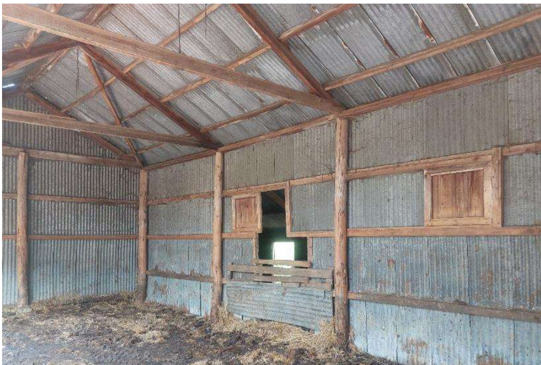
Figure 17 The interior of the modern shed to the south-east of the L-plan range of buildings.
