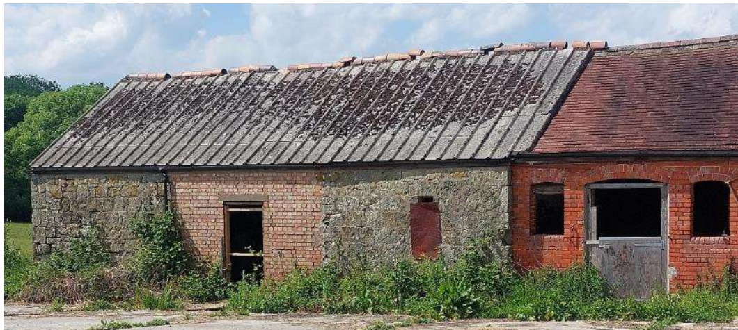
Figure 6 The stone-built barn at the west end of the L-plan range, south elevation.
