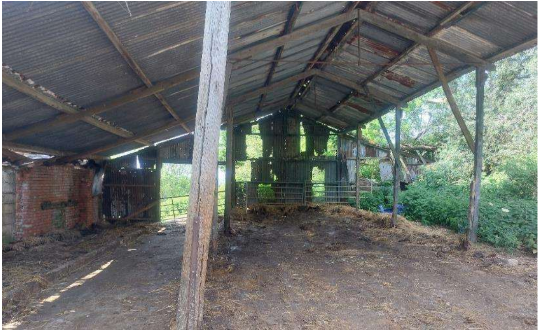
Figure 16 The modern agricultural shed attached to the east side of the L-plan range, facing north.
