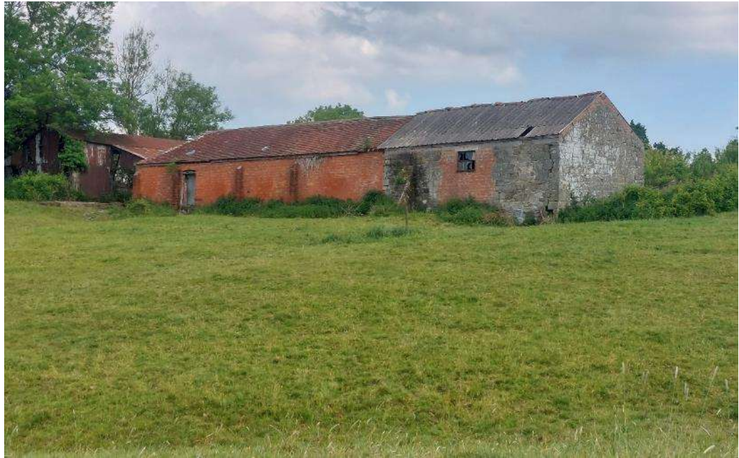
Figure 22 Viewpoint 4: A view to the north elevation of the L-plan range from the public footpath moving closer to the buildings.
