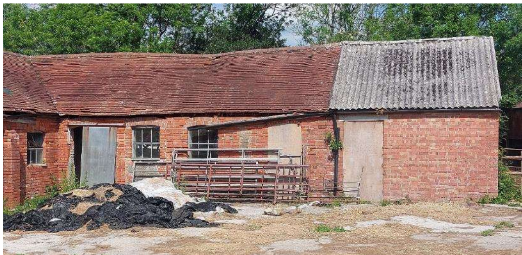
Figure 10 The return of the L-plan cow shed range, west elevation showing the two phases of construction marked by the change in roofing material and brickwork.
