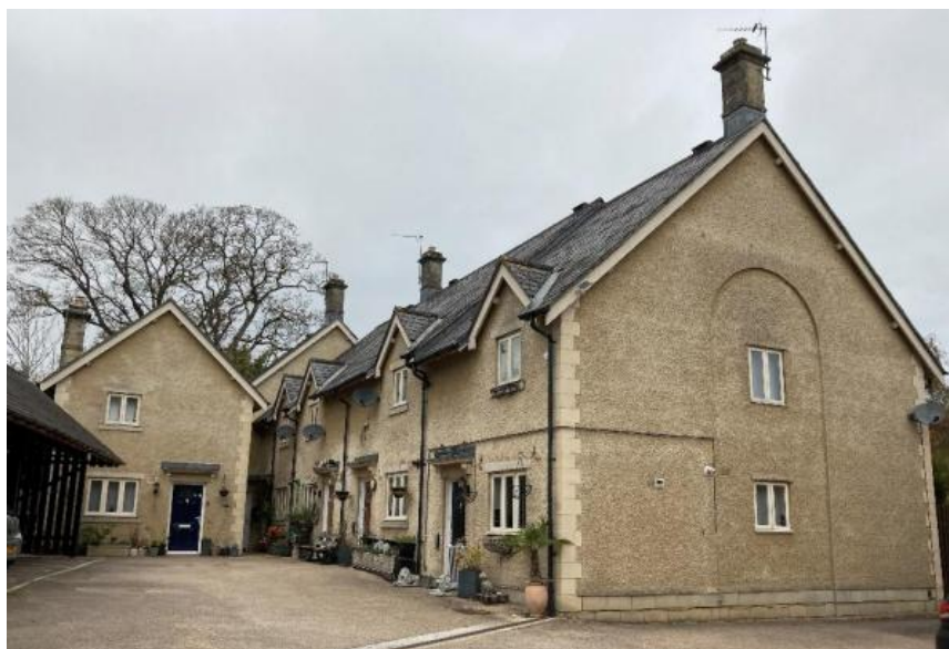
Figure 4: view of site from west, showing existing materials (from heritage statement)
