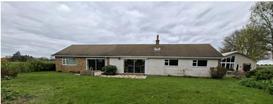
Figure 1: Showing outdated and disjointed appearance of 'Canfield' from within site to its south.
