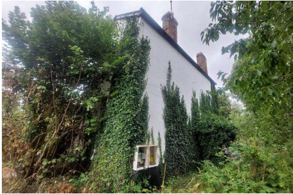
Figure 5 The rear elevation of Gas Cottage.
