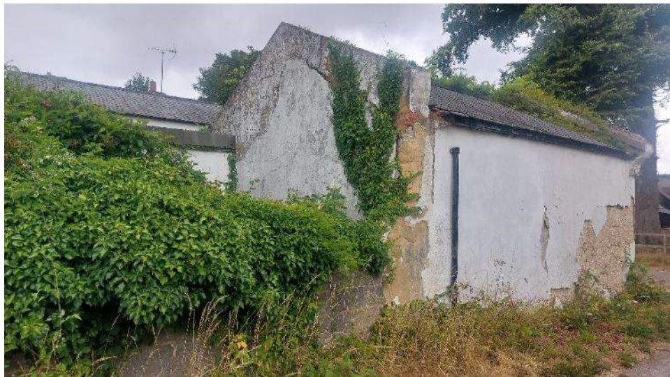
Figure 8 Ancillary building, west and south elevations.
