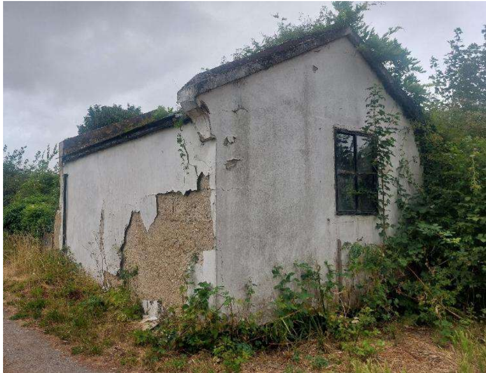
Figure 7 Ancillary building, south and east elevations.
