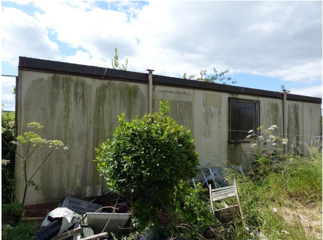
Figure 21: Northern aspect of Portakabin
