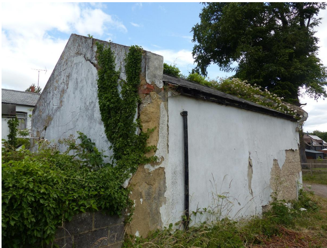
Figure 17: Slate tiled roof & ridge of the Outbuilding
