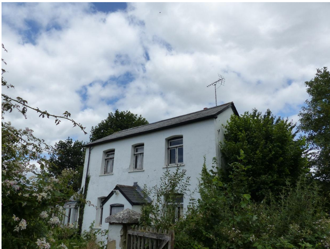
Figure 7: Southern and eastern aspects of Gas Cottage
