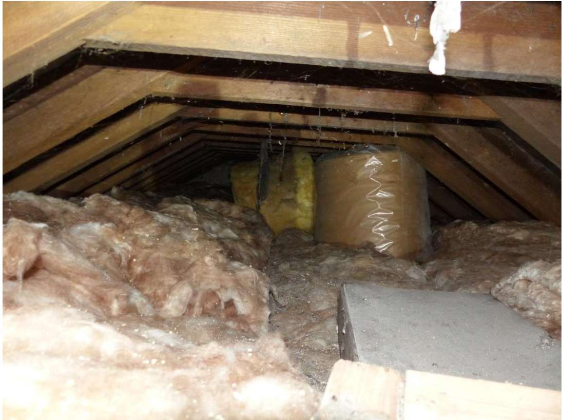
Figure 14: Void space viewed eastwards from access hatch
