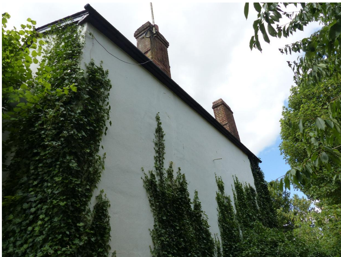
Figure 8: Northern aspect of Gas Cottage
