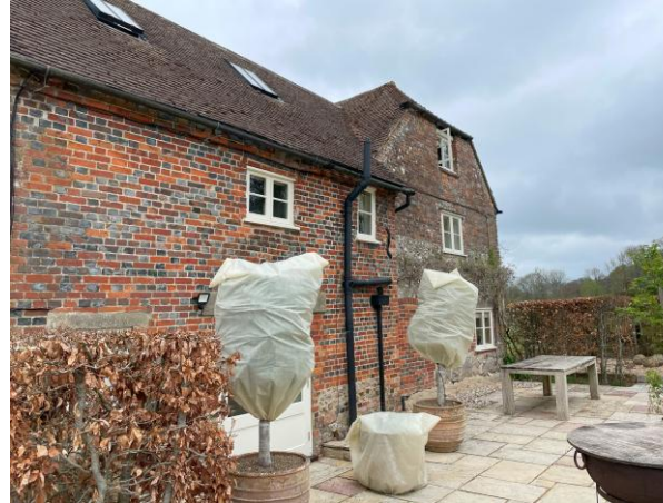
Farmhouse southeast elevation
