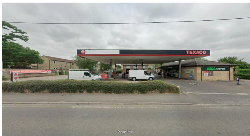
Figure 6: Street view (Google, 2024) of site from Pickwick road
