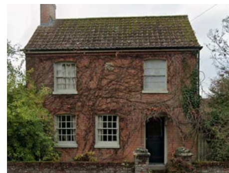
Brick arches, eight over eight sash windows
