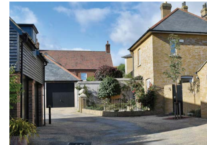
Figure 56: Example photograph of a CG Fry courtyard in Poundbury
