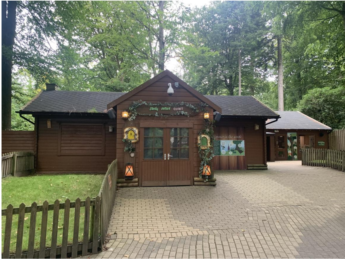
Figure 4: Existing Grotto building (Structure A).
