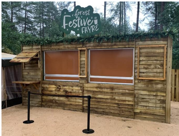
Figure One (left): Precedent Image of Temporary Food & Beverage Kiosk building at Sherwood.
