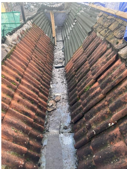
Valley showing lead gutter and pantile and slates in same roof pitch.
