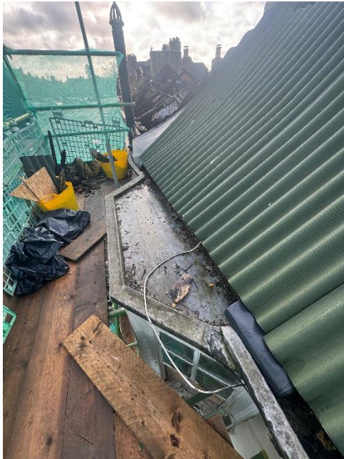
Flat lead roof with shallow upstand
