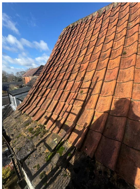
Traditional pantile roof – out of scope of repair
