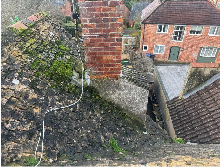
Swept tiles to valley
