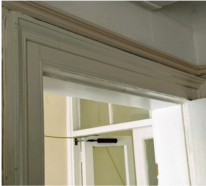
Fig.34 6-panel door to Family room Fig.35 Ogee-moulded architrave surround
