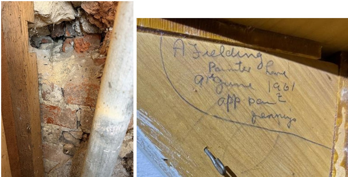
Fig.68 Fireplace return seen in stair cupboard. Note stonework perhaps for an ashlar lintel, and smoke blackening
