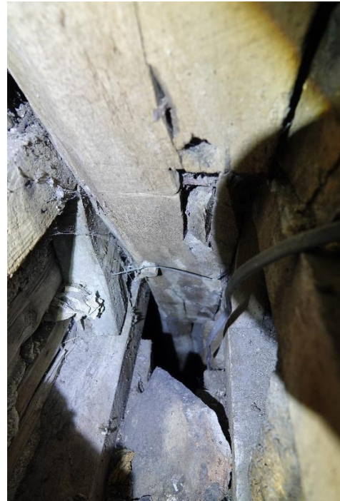
Figs. 95 & 96. Truss T2, showing (left) the mortise for a lost collar; (right) further vacant mortises glimpsed inside the lath-and-plaster partition
