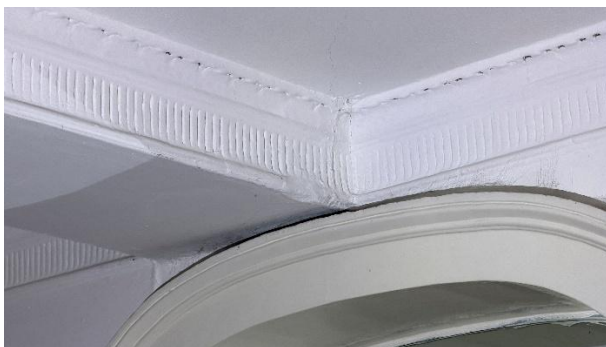
Fig.33 Detail of deeply-overpainted acanthus cornice with ribbed frieze. Note ogee-moulded and flat architrave surround of central wall recess
