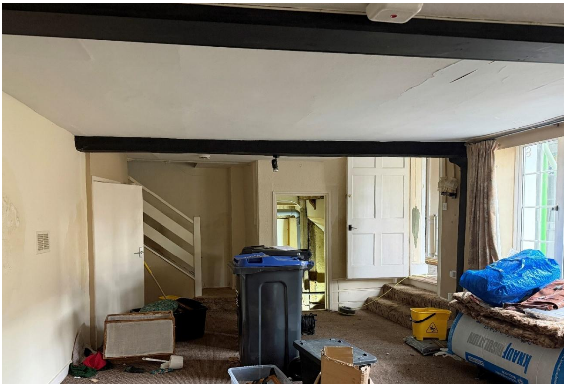
Fig.65 Blocked kitchen fireplace (left), c1960 stair, cellar entrance and 6-panel door on HL hinges
