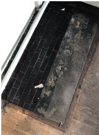
Fig.39 C1900 tiling to c1800 hearth Fig.40 Moulded cornice and plastered beam
