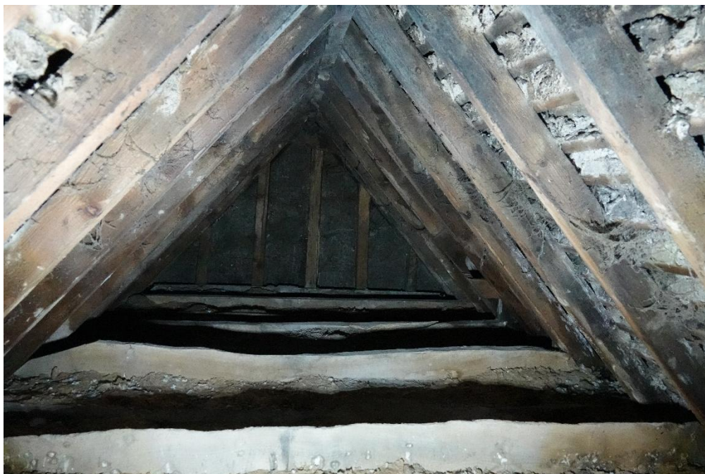
Fig. 103. The roof of the rear wing (bedroom 2)
