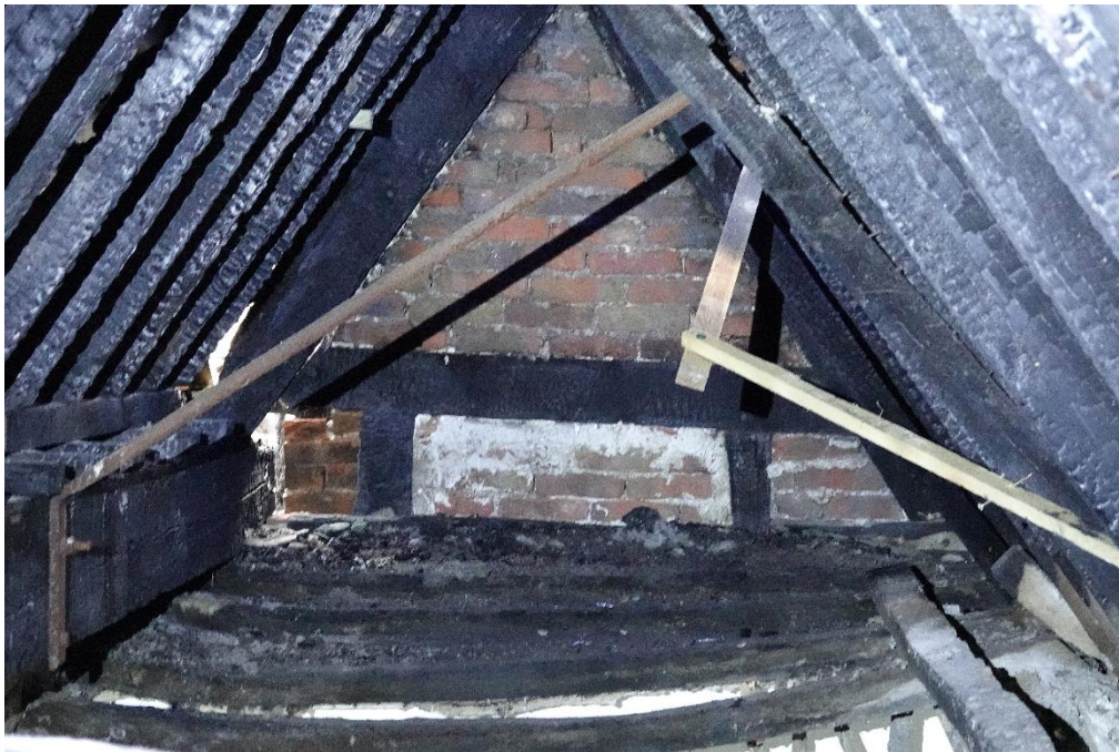
Fig.84. Truss T1 as seen from the loft hatch
