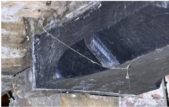
Figs. 12 & 13 17 th century concave stop with roll moulding at Studley Grange Farm, Lydiard Tregoze. A similar moulding appears to have been removed from the rear range ground floor beam at 3 Northgate Street
