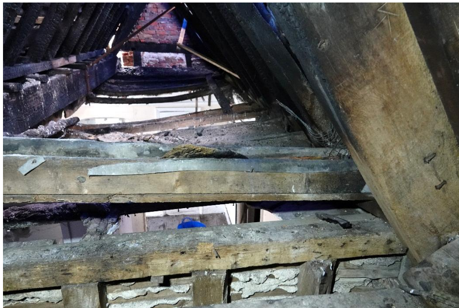
Fig. 97. The lead-lined gutter cutting through the roof space by T2
