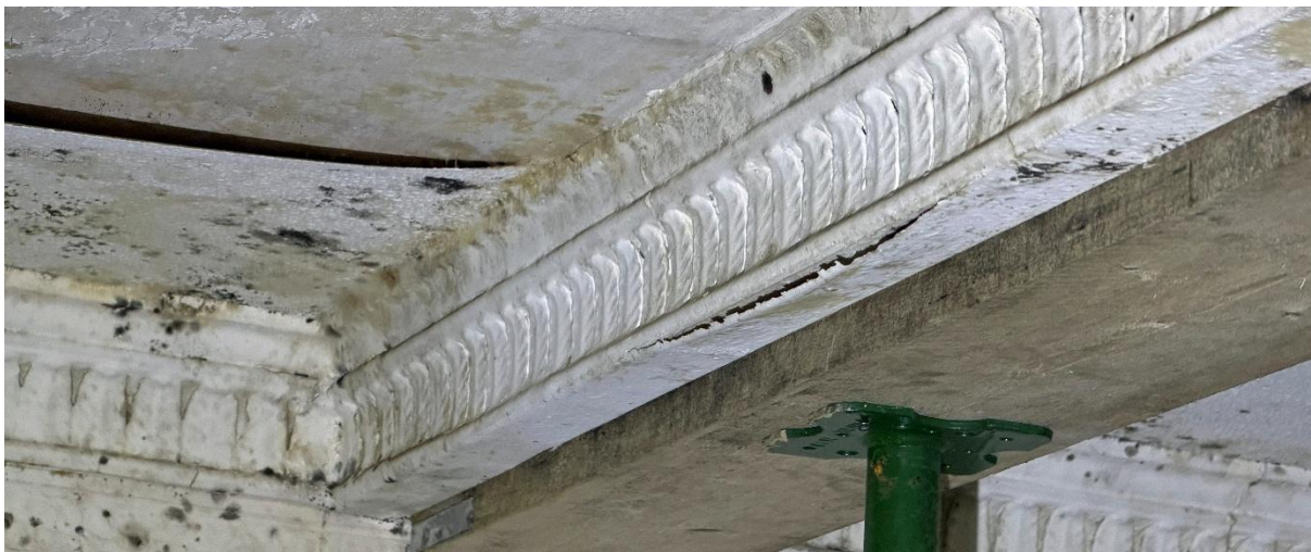
Fig.29 Continuation of moulding along beam
