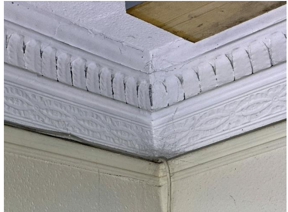
Fig.28 Detail of cornice
