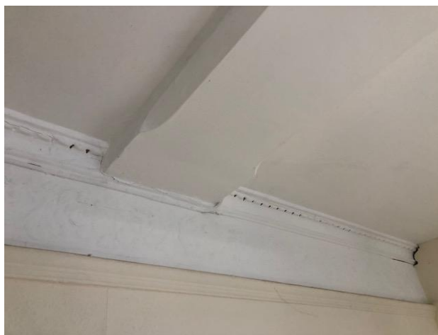
Fig.39 C1900 tiling to c1800 hearth Fig.40 Moulded cornice and plastered beam
