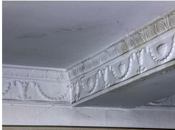
Fig.51 Detail of egg-and-dart moulding, with swagged frieze
