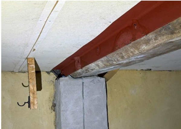
Fig.82 Reused 17 th century beam in cellar
