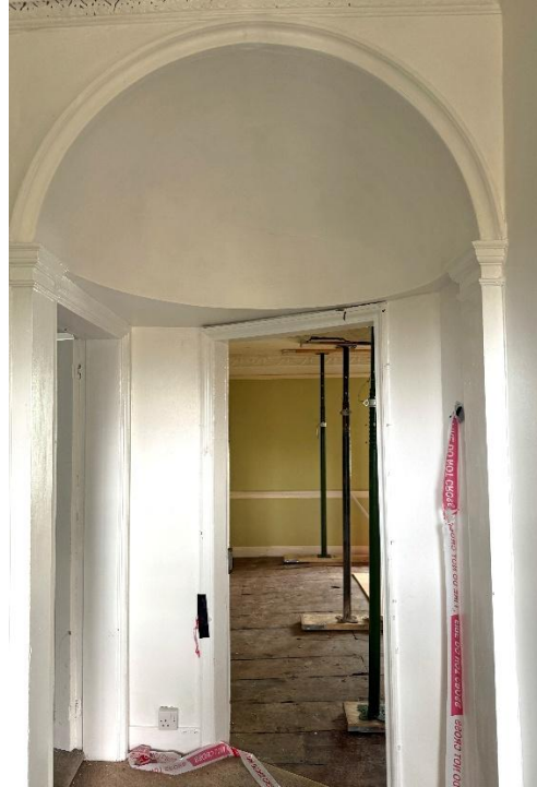
Fig.43 Half dome over lobby to front bedrooms
