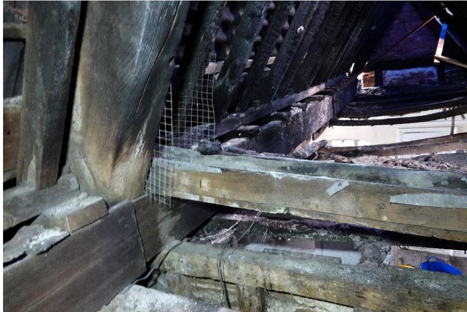
Figs. 91. Truss T2, showing on the left the principal rafter of the front slope. The internal gutter can be seen cutting across the centre of the image, and below it, the top of a framed lath-and-plaster partition. See also Fig. 97.
