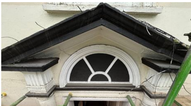
Fig.17 Semi-circular false fanlight in open pediment
