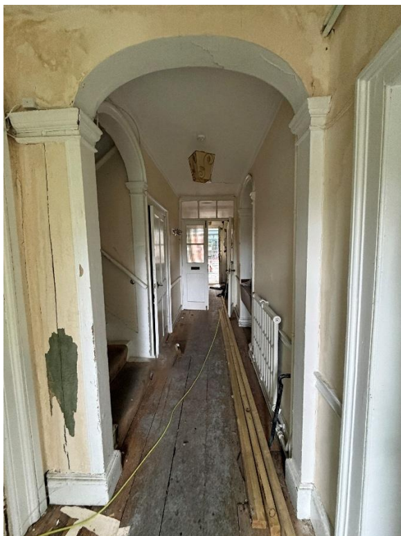
Fig.24 Hall looking towards front door. Note the stilted segmental arches with moulded imposts. The closest arch may have lost its moulded architrave surround. The glazed double doors with overlight is circa 1900
