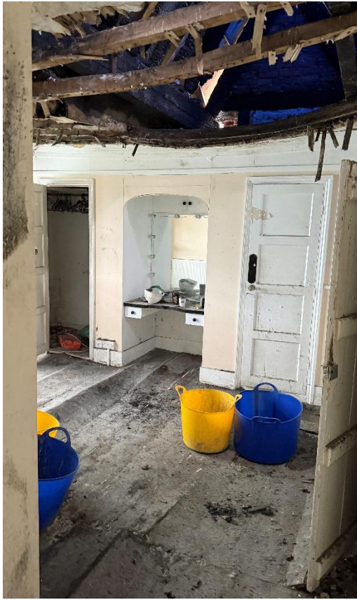
Fig.63 South Attic Room from doorway
