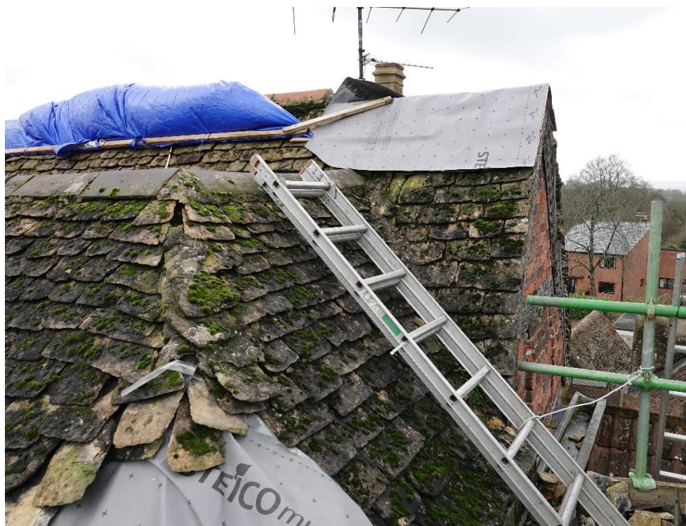
Fig. 90. The roof the subsidiary front roof in relation to that of the main range
