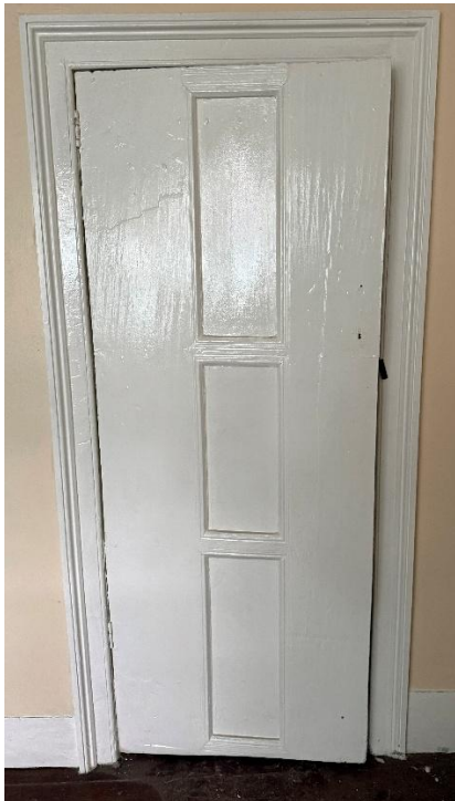
Figs.61 & 62 Outer and inner skins of later 17 th century door
