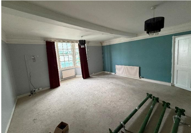
Fig.45 Plastered beam and acanthus cornice as on the ground floor
