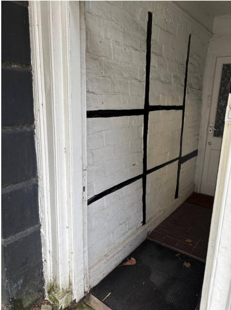
Fig.19 Light timber-framing of c1800 with edge-set brickwork panels forming the north return
