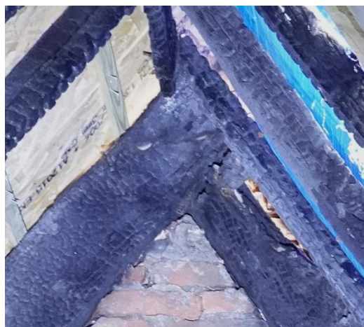
Fig. 85. The apex of Truss T1
