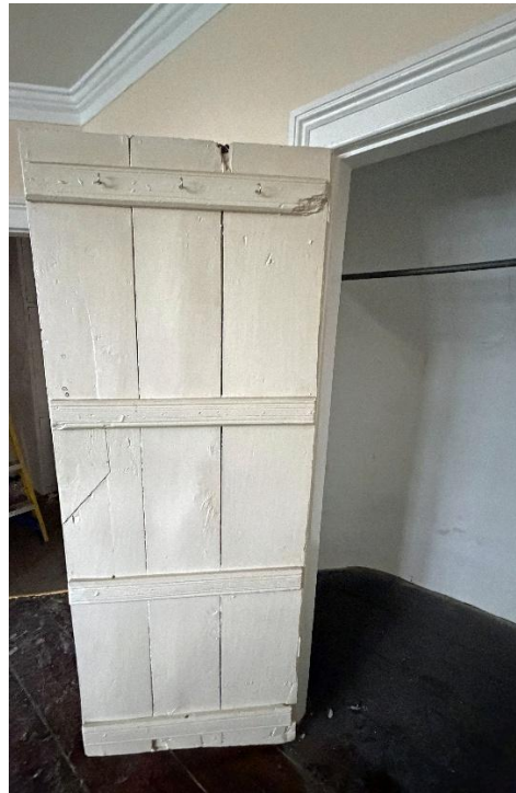
Figs.61 & 62 Outer and inner skins of later 17 th century door
