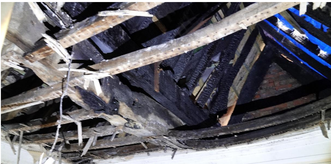
Fig. 87 View from the ceiling of the bedroom below
