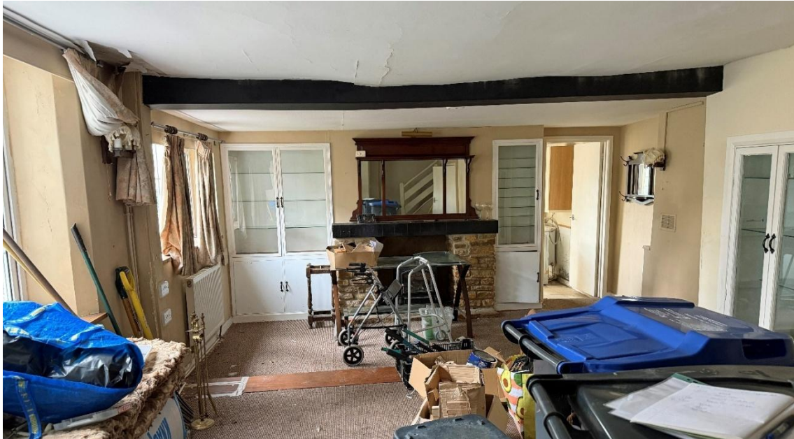
Fig.64 Sitting Room looking west to false fireplace. A partition wall was at the step down and the beam above may be a boxed steel
