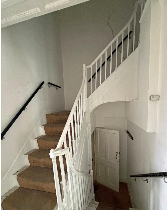
Fig.42 Stair from ground floor
