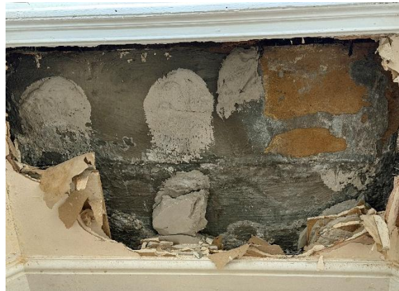
Fig.32 Ashlar stonework inside bay
