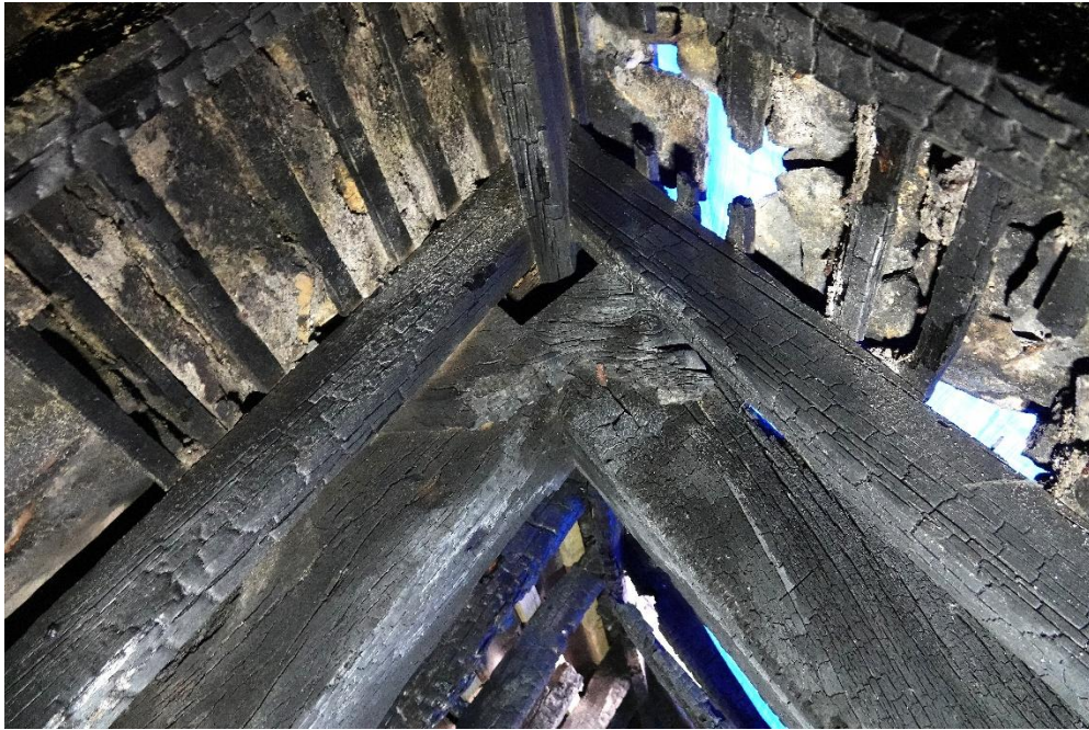
Fig. 93. Truss T2, apex detail
