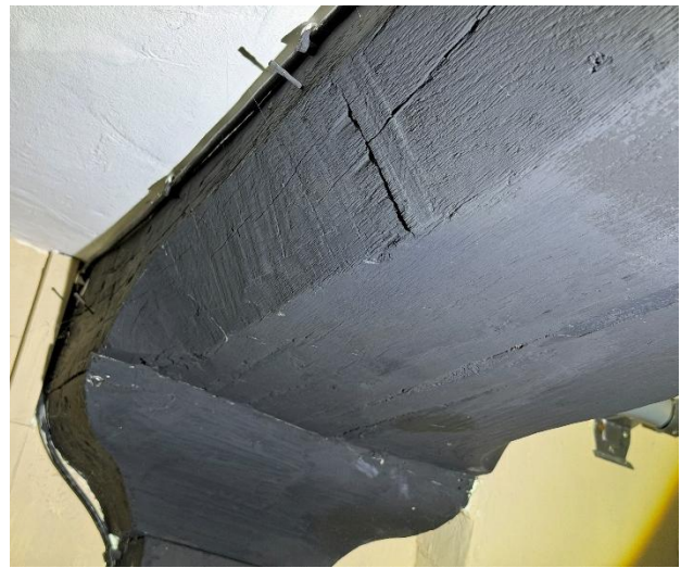
Figs. 12 & 13 17 th century concave stop with roll moulding at Studley Grange Farm, Lydiard Tregoze. A similar moulding appears to have been removed from the rear range ground floor beam at 3 Northgate Street
