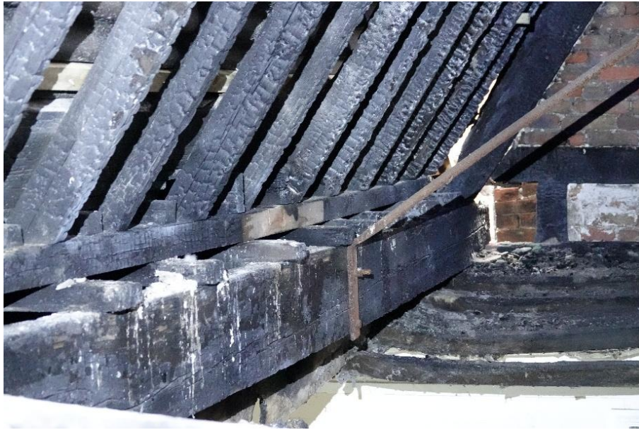
Fig. 86. The horizontal plate in bay T1-T2
