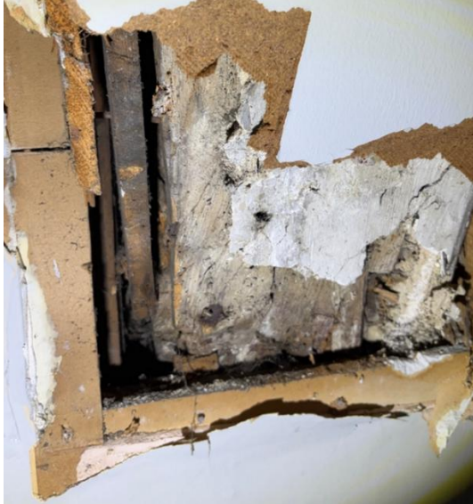
Fig.70 Nailed bracket to tie-beam on north wall at first floor level
