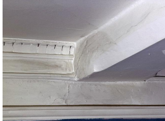
Fig.45 Plastered beam and acanthus cornice as on the ground floor
