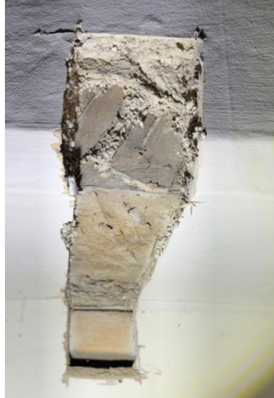
Fig.70 Nailed bracket to tie-beam on north wall at first floor level
