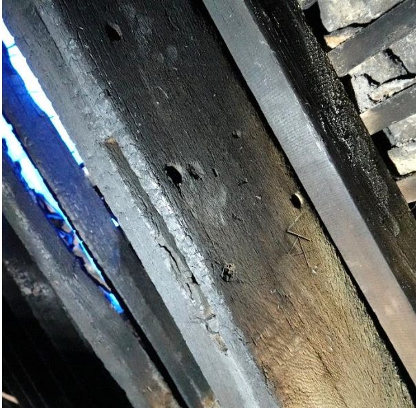
Figs. 95 & 96. Truss T2, showing (left) the mortise for a lost collar; (right) further vacant mortises glimpsed inside the lath-and-plaster partition
