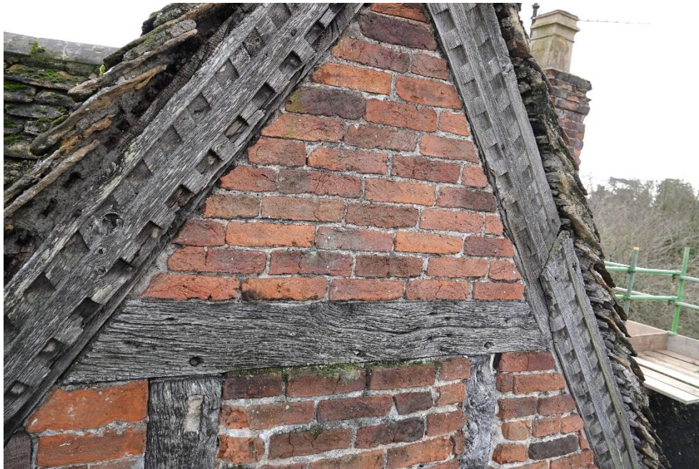
Fig. 100. Truss T3 and the timber-framing of the end wall
