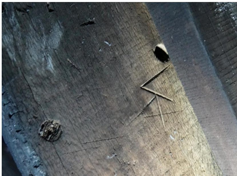
Fig. 94. Truss T2, carpenter's mark
