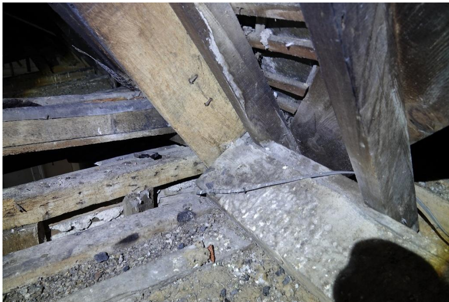
Fig. 92. Truss T2, showing the principal rafter on the rear slope
