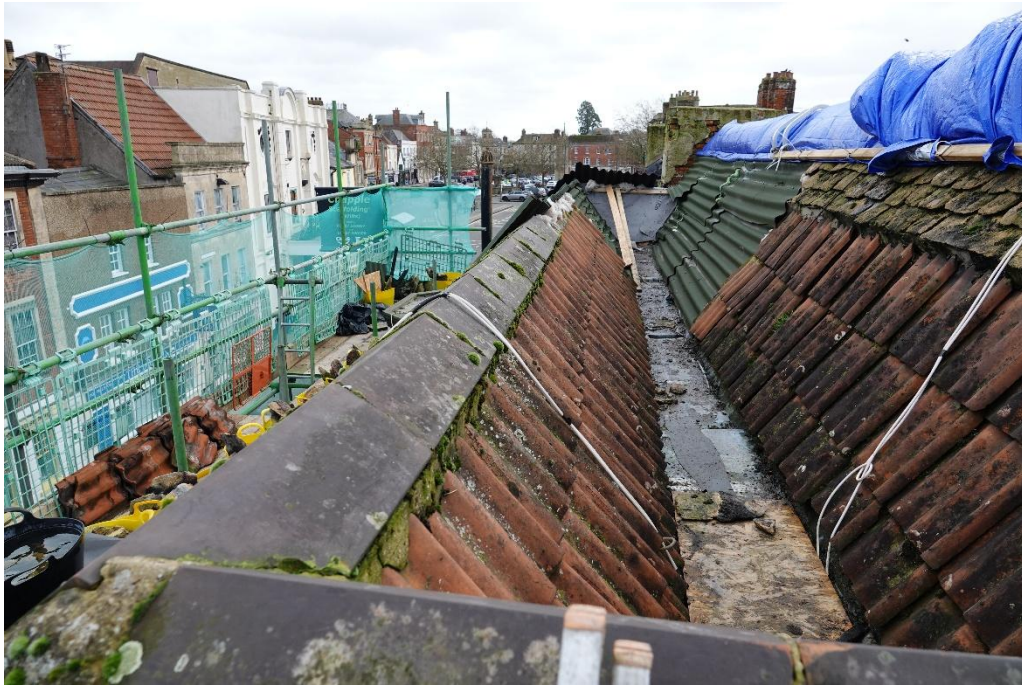
Fig. 89. View looking SE showing the subsidiary front roof
