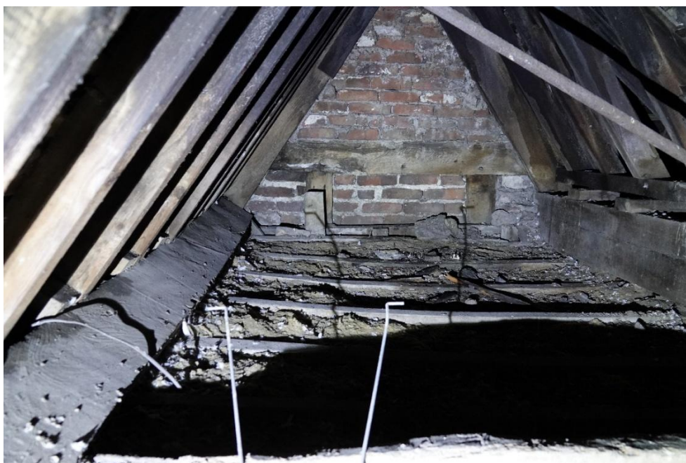
Fig. 98. A general view of bay T2-T3 and Truss T3
