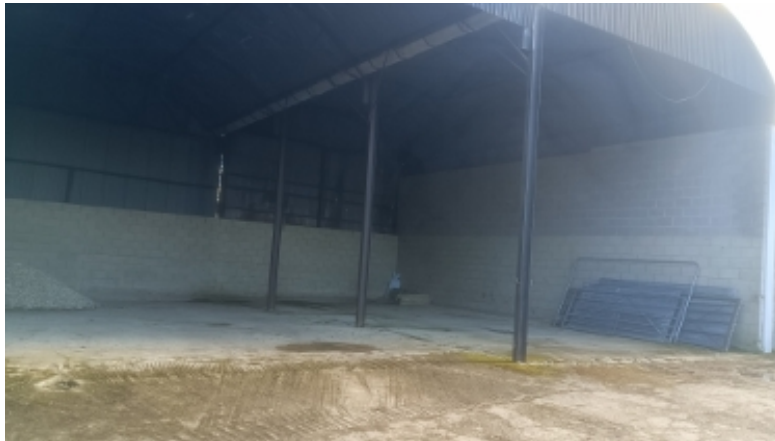
Photo 8. Interior of steel framed barn / building B
