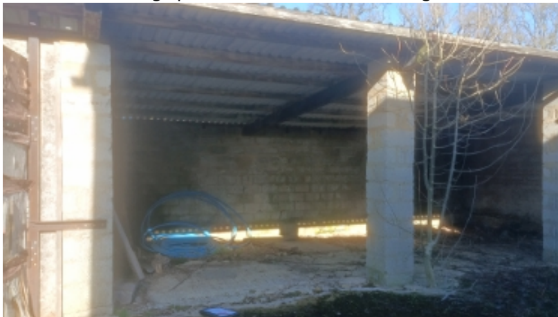
Photos 5. Showing open fronted section of building C
