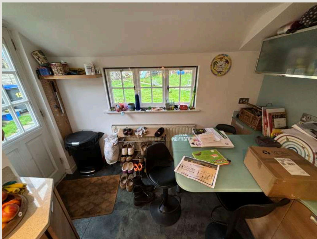
Image 04 / Ground floor kitchen. Non-original windows in triple bay arrangement as opposed to the existing cottage twin style which is predominant on the South elevation.
