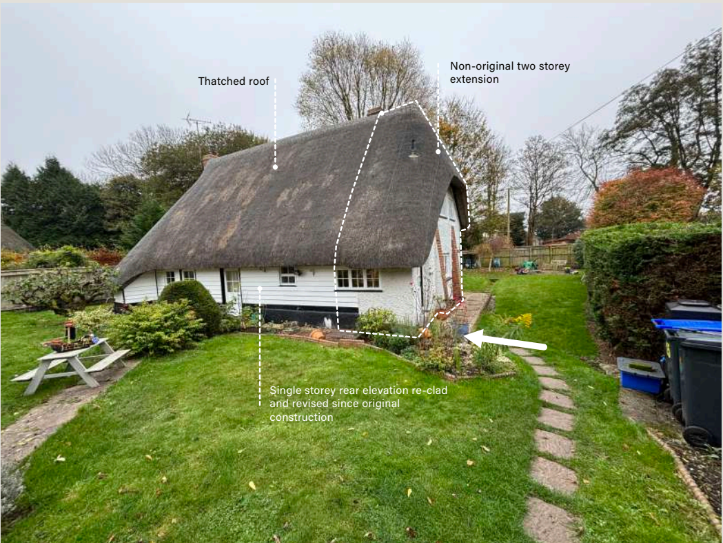
Image 04 / View from the North and modern entrance side of the plot. The existing kitchen side door currently operating as the main front door to the house.
