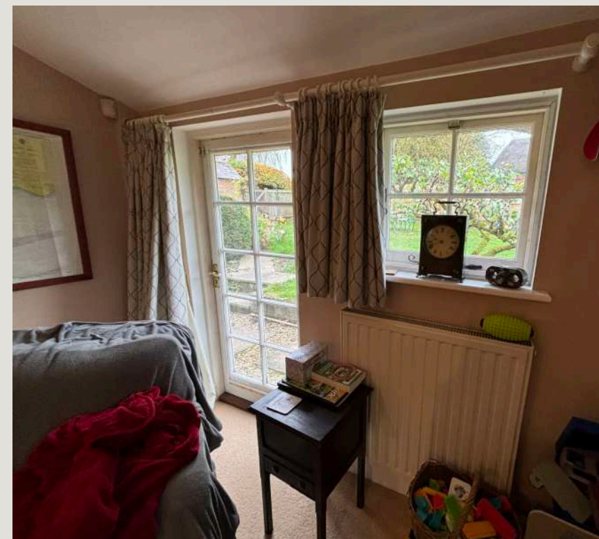
Image 04 / Ground floor living space. Non-original window & door to North elevation. Modern radiator to existing wall.
