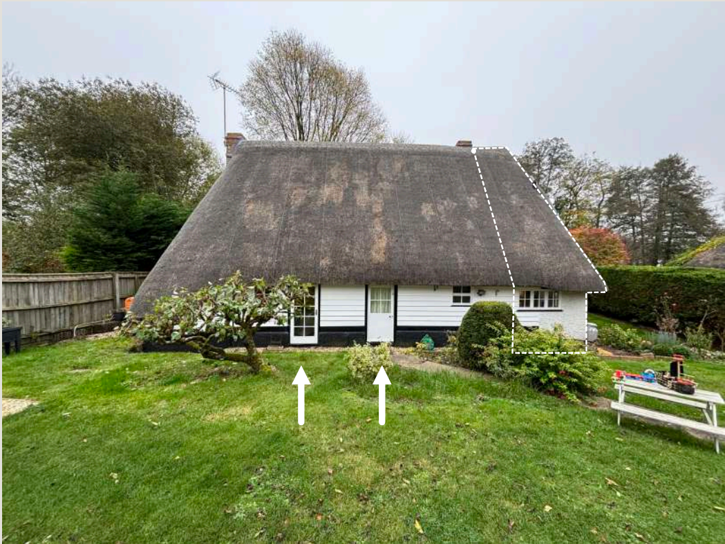
Image 03 / View from the North rear garden at the primarily non-original catslide type rear roof and painted weatherboard cladding.
