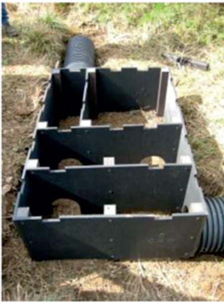
Otter holt assembled and installed before lid is attached.
