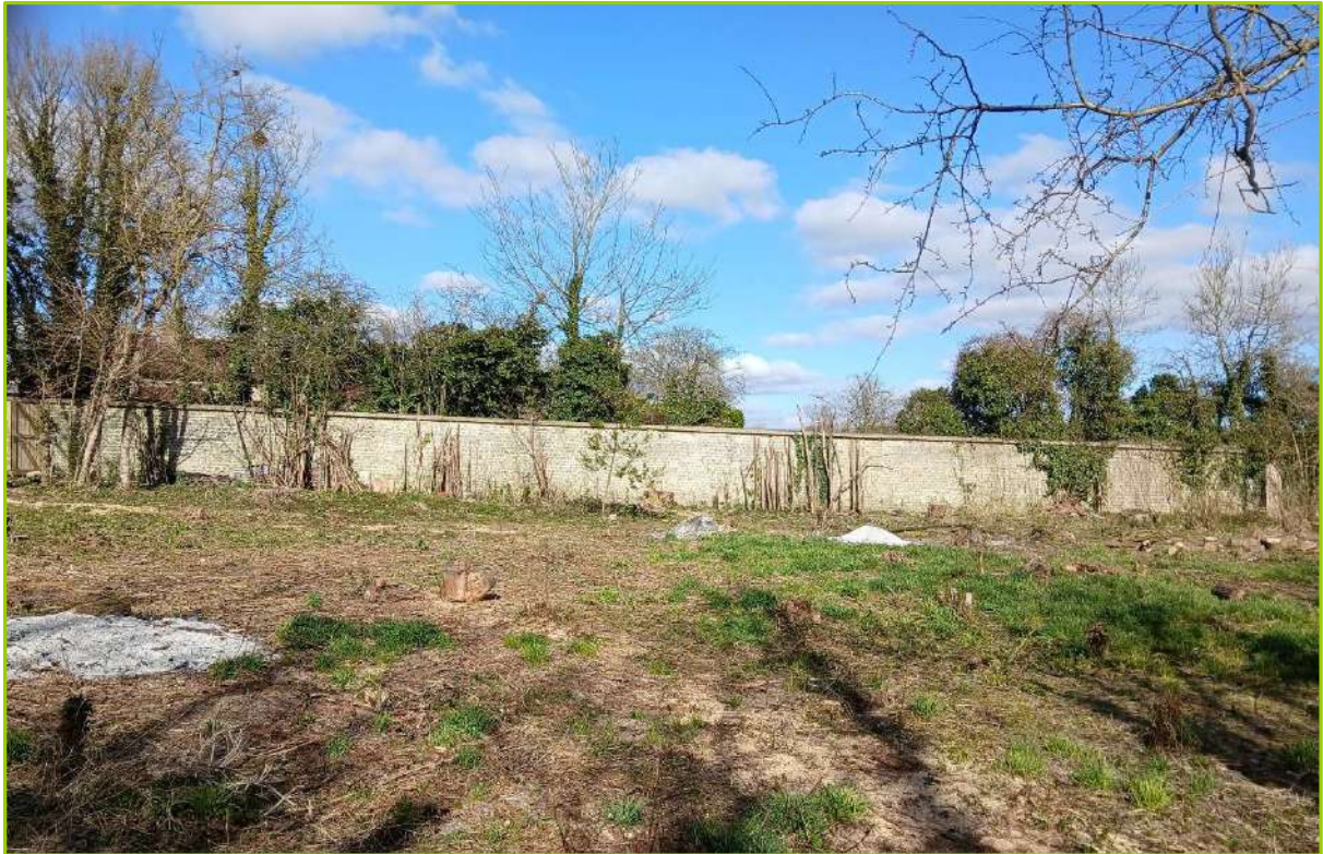
Photo 2 - View looking North
