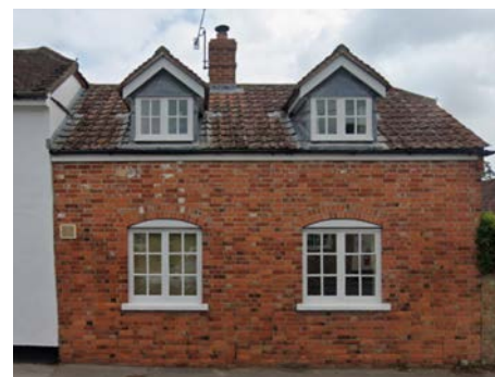
Brick arches, casement windows, brick arches, tile roofs
