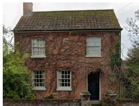
Brick arches, eight over eight sash windows
