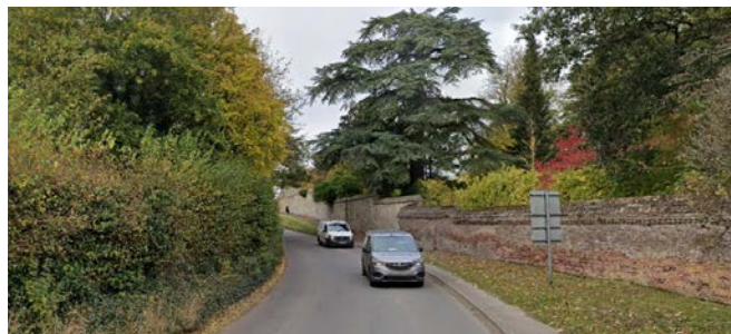
Figure 38: The Manor, West Lavington, high stone wall. (Google Street View)
