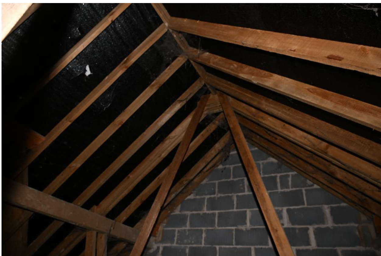
Image 4 Roof structure Image
