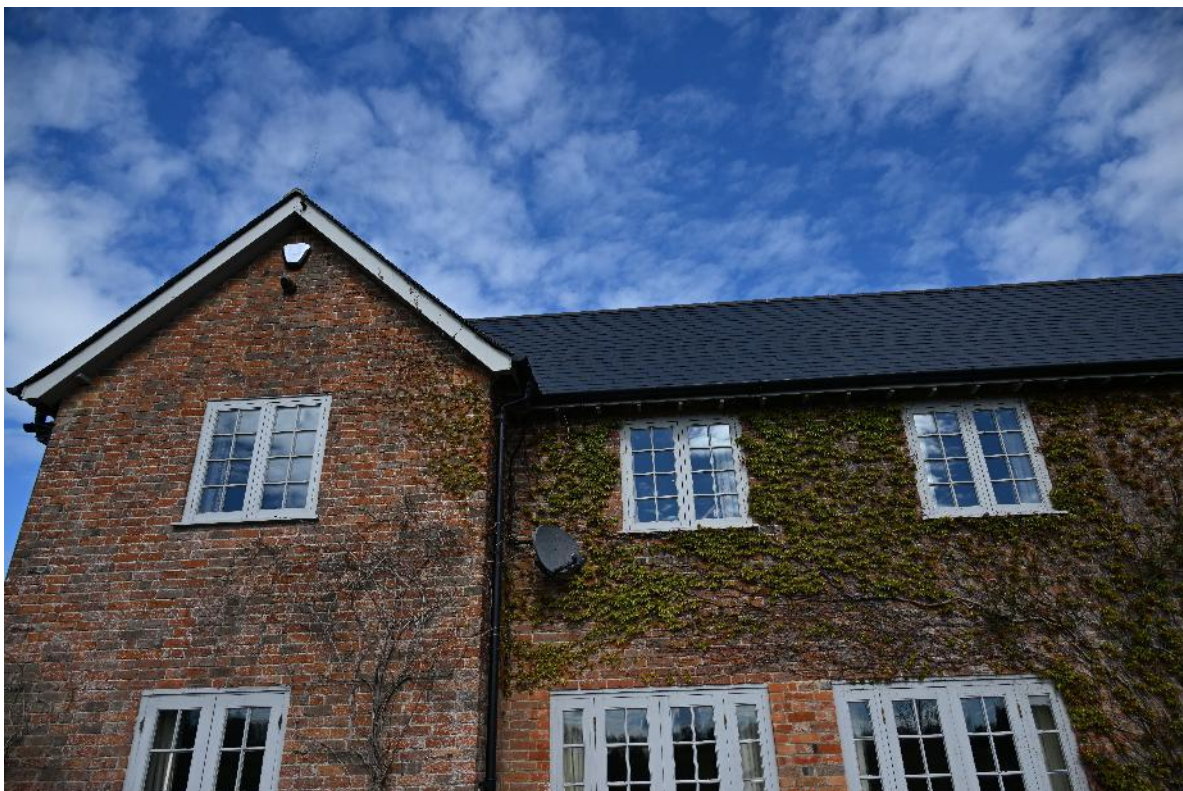
Image 2 Well appointed building with a lack of PRFs
