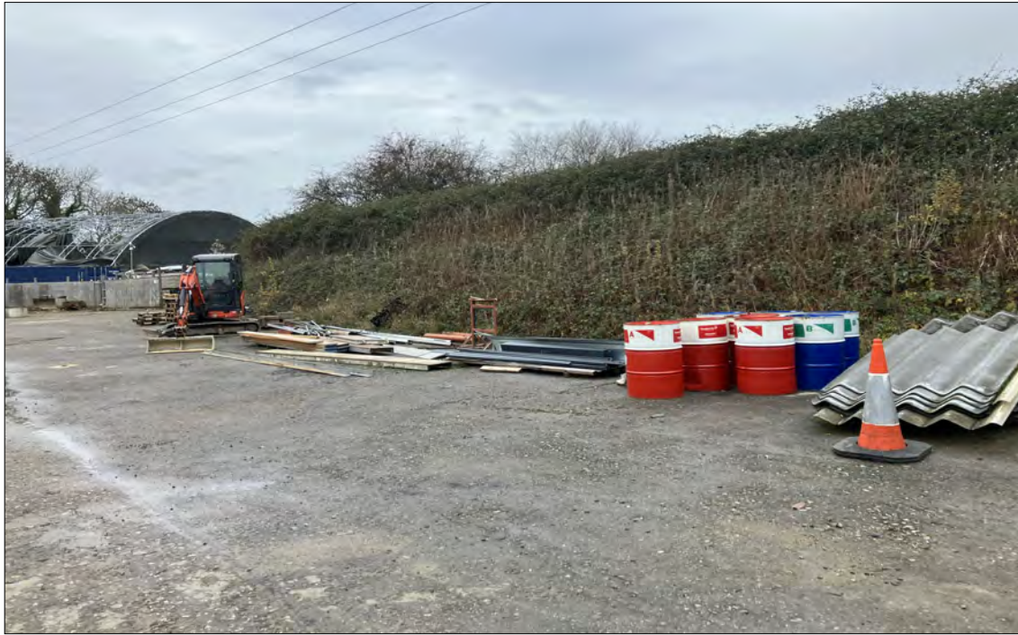
View north - laydown area to east of main commercial unit
