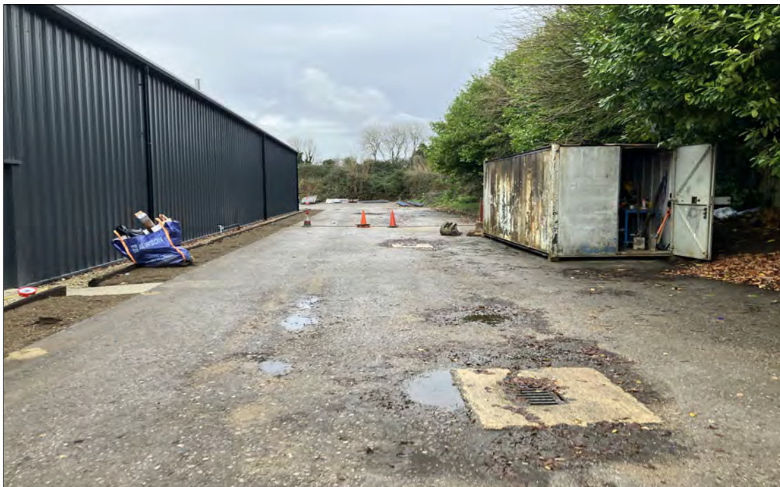
View east - access and laydown to south of main commercial unit
