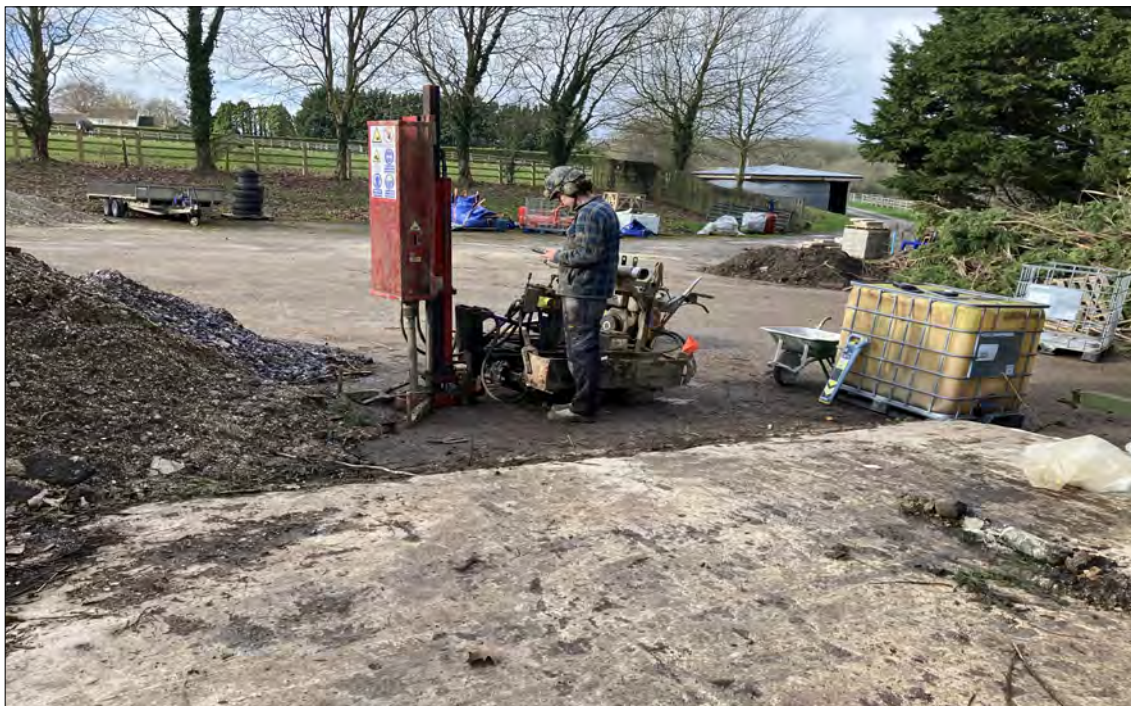
Drilling at WS02A
