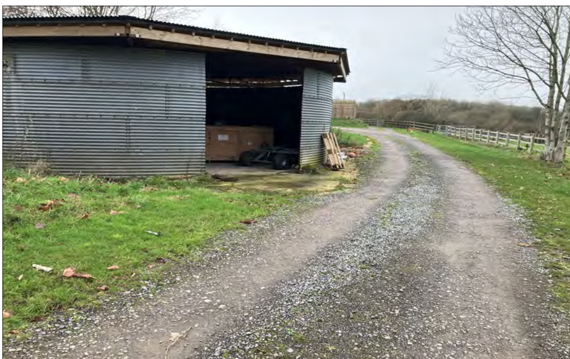
View west - old pumping and storage shed
