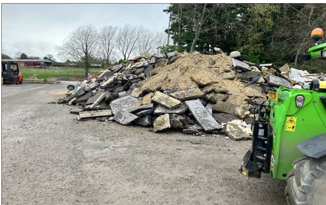
Stock piled demolition waste in laydown area
