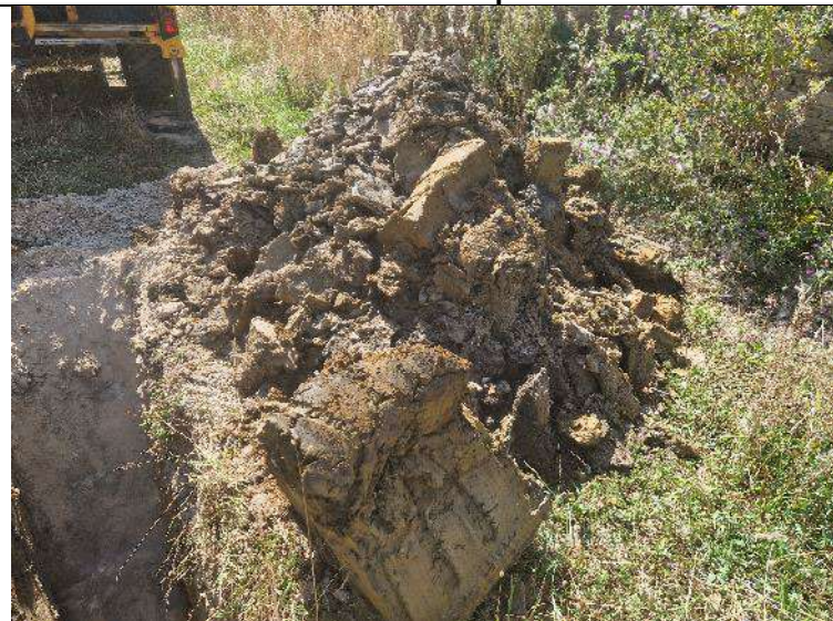
PLATE 12 – Trial Pit Spoil – TP03.
