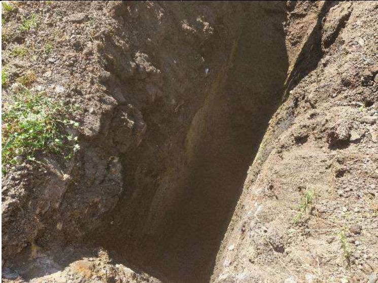
PLATE 13 – Trial Pit Excavation – TP04.
