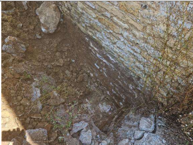
PLATE 21 – Trial Pit Excavation – FP05.
