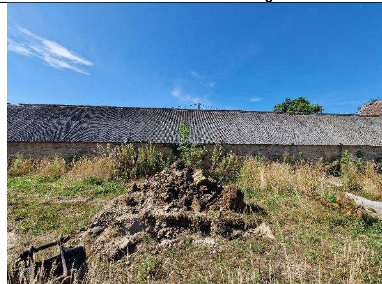
PLATE 04 – Site Overview – Looking South.
