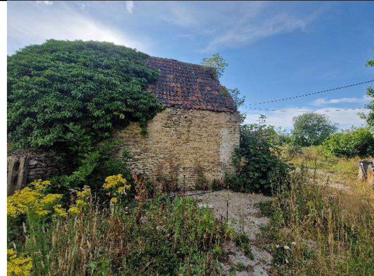
PLATE 02 – Site Overview – Looking South East.
