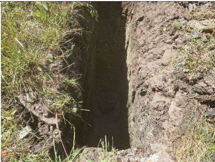
PLATE 15 – Trial Pit Excavation – TP05.
