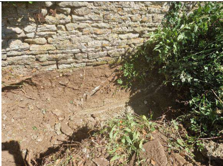
PLATE 17 – Trial Pit Excavation – FP01.
