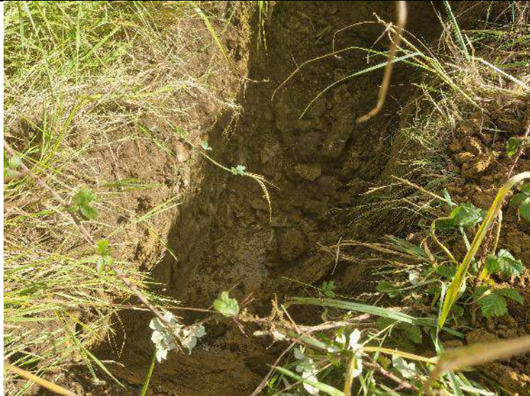
PLATE 09 – Trial Pit Excavation – TP02.
