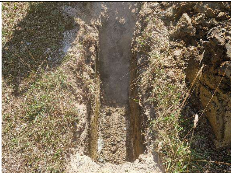
PLATE 11 – Trial Pit Excavation – TP03.
