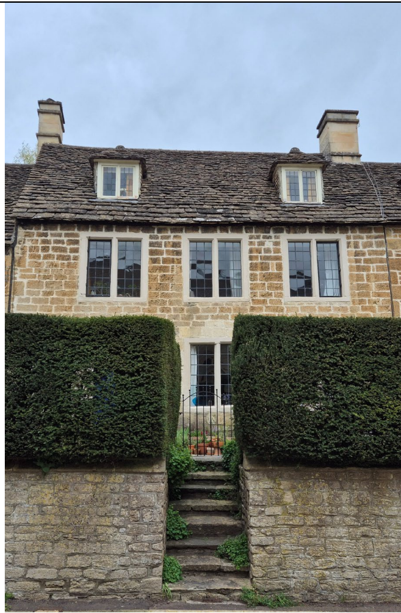
Fig 2: No.11 Church St from the road
