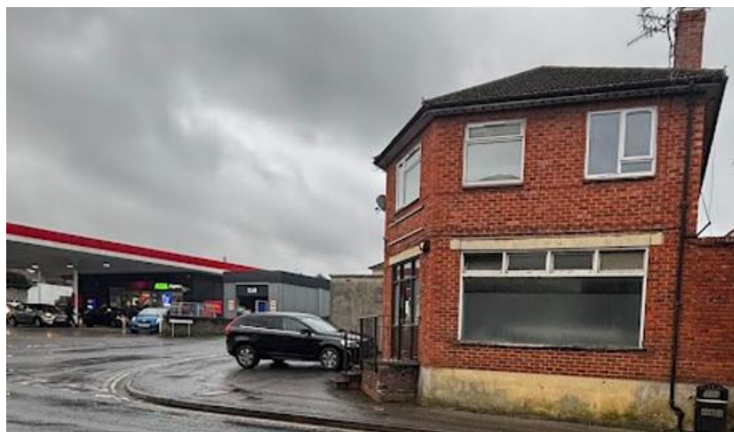
Proximity of the petrol station located to the southeast of the building
