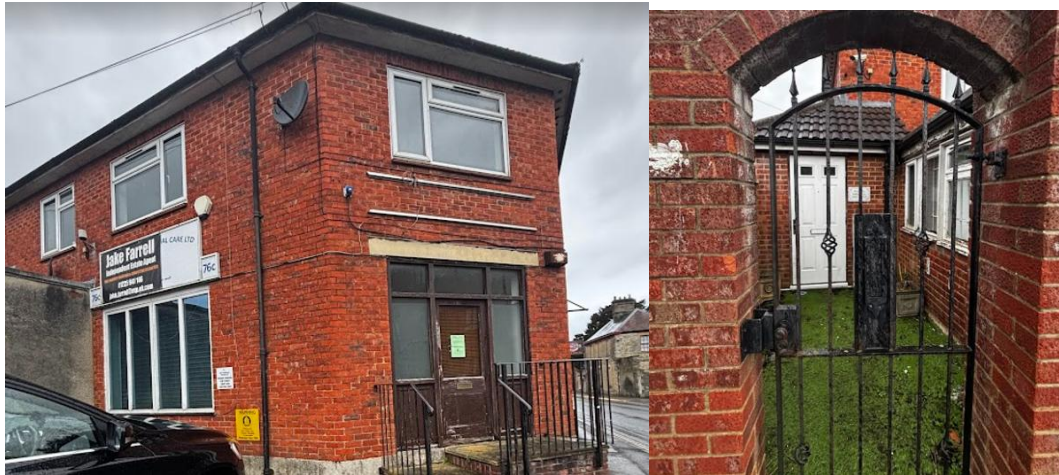
Front (northeast) elevation and side (southeast) elevation
