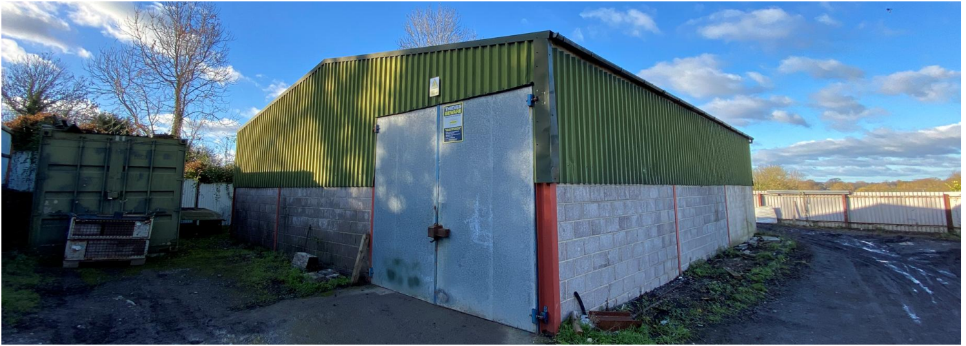
Site Visit South Elevation
