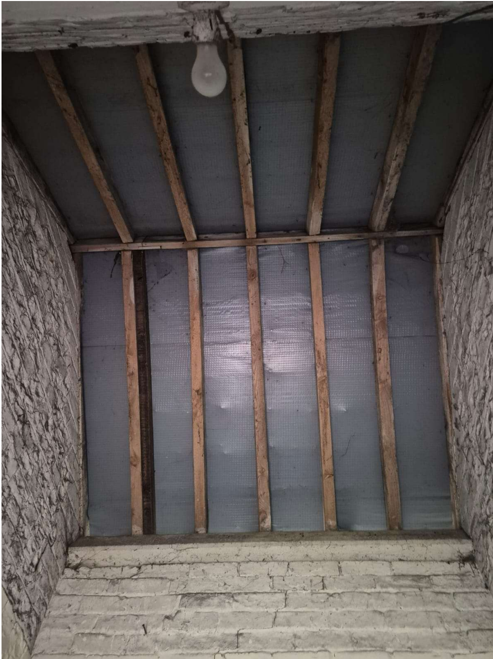
Image 4: Roof space of the storage cupboard
