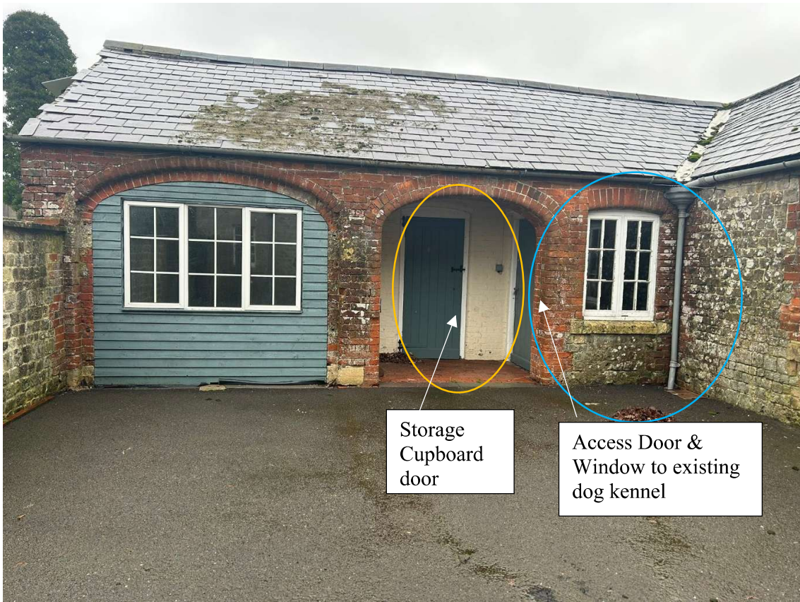
Image 2: Existing Dog kennel access & window and storage cupboard door.
