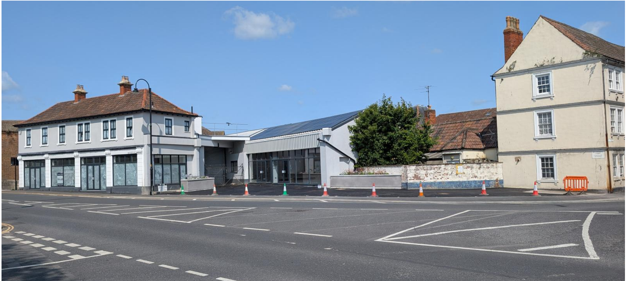
Photo 1: Existing view of application site. The proposed roof level condenser units will not be visible from this viewpoint or elsewhere in the public domain.
