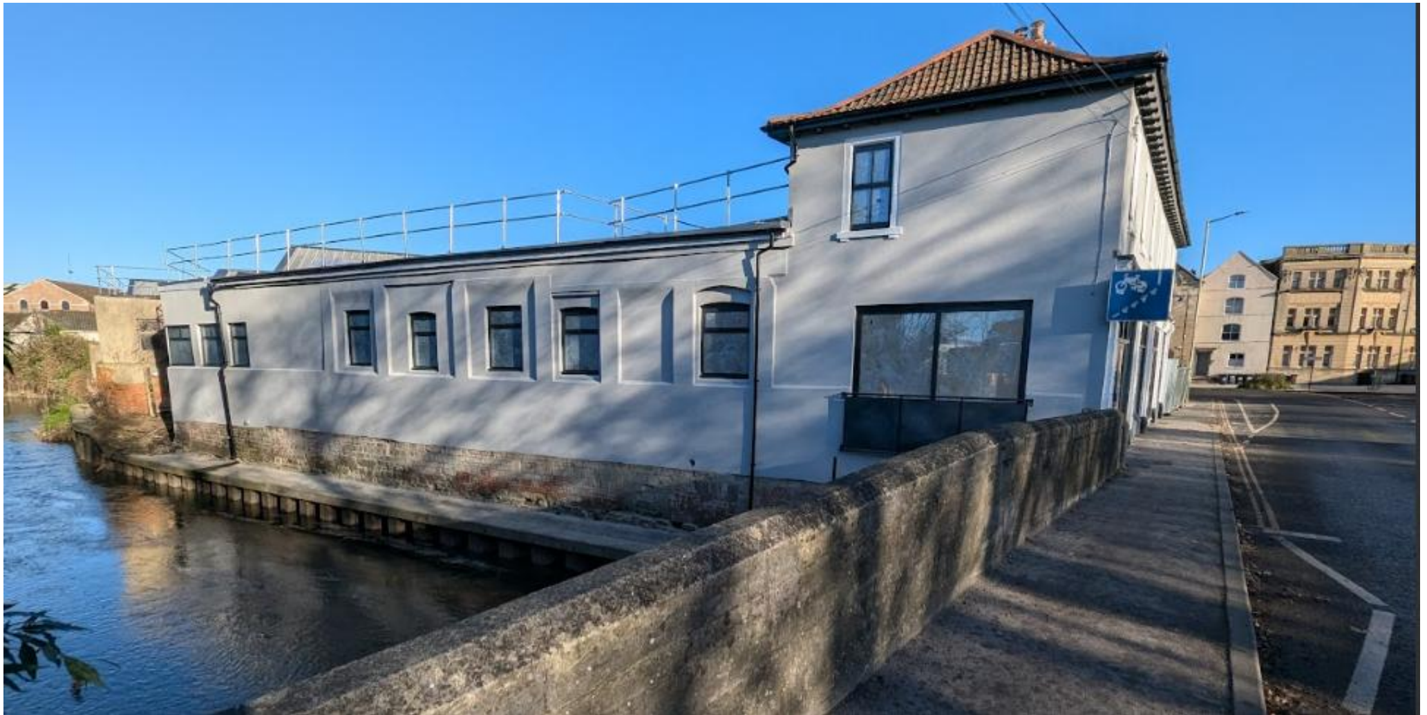
Photo 2: Existing view of application site. The proposed roof level condenser units will not be visible from this viewpoint or elsewhere in the public domain.
