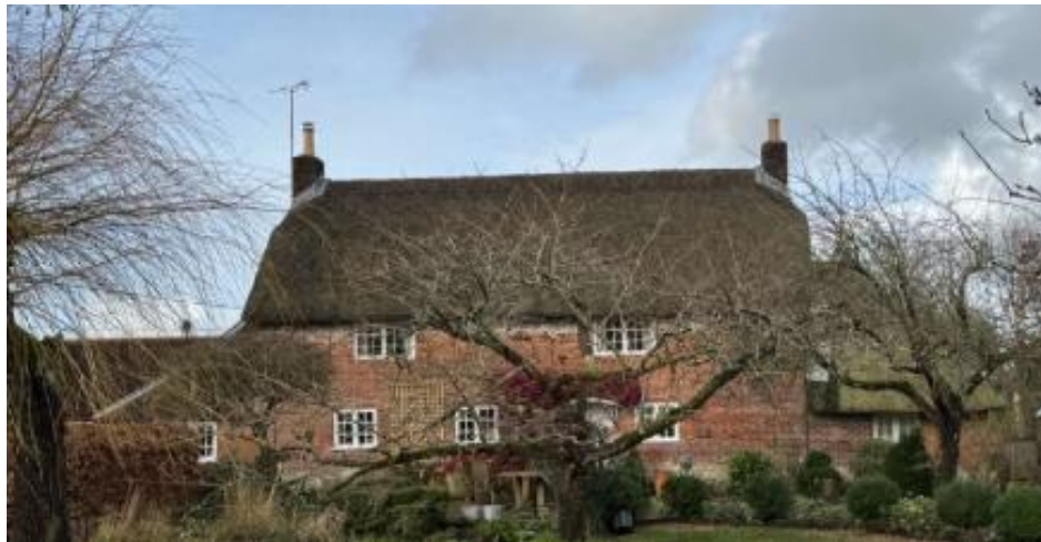
Photo of the existing chimney arrangement
