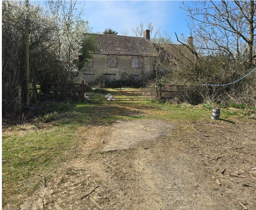
Photo 10: A view of the old farmhouse
