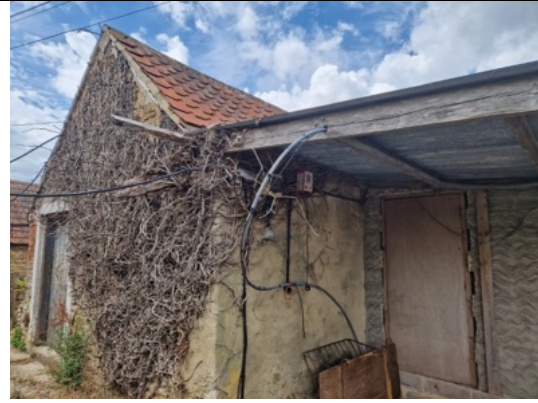
Photo 15. South elevation of B4
