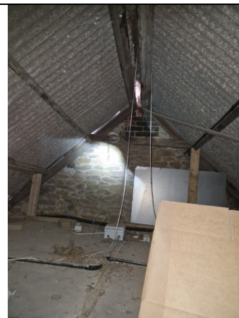
Photo 18. Interior North end B4
