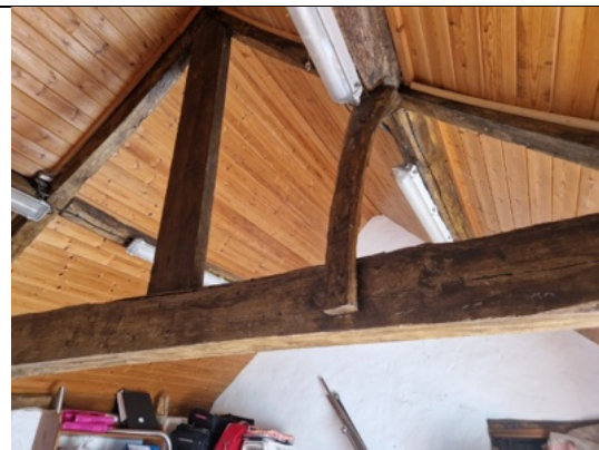
Photo 17. Attic room South end B4
