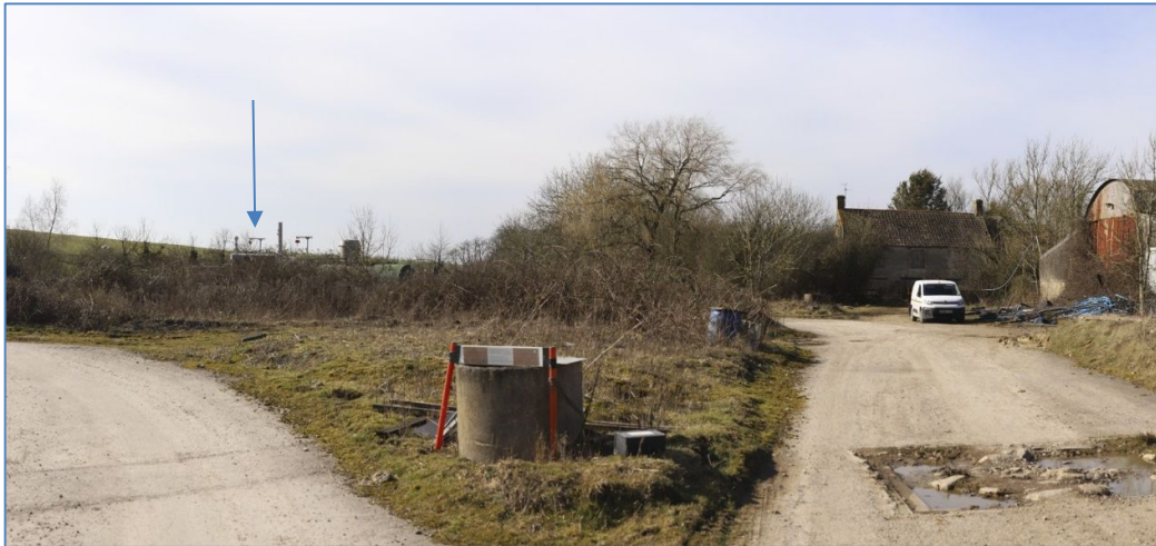
Figure 17 View west looking to front elevation of Studley Grange and to the left the existing gas installation (arrowed).
