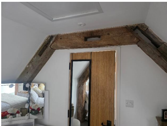
25 – Existing Truss retained with partition and door set behind to form Ensuite
