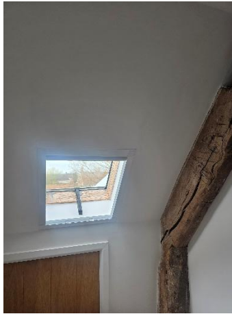
11 – Rooflight & Door to Eaves Storage
