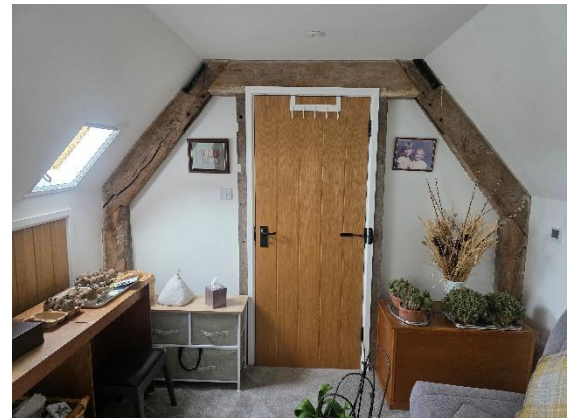
26 – Existing Truss retained with partition and door set behind to form Stair landing
