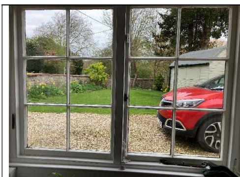
Window W2 internally
