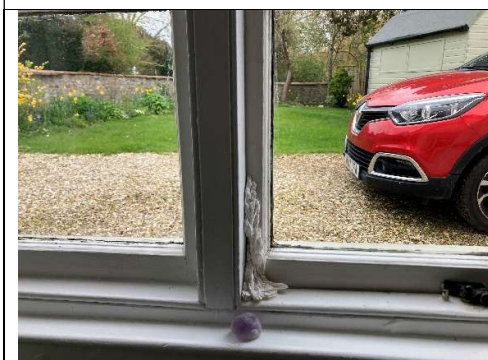
Note tissue paper to seal up hole in casement frame
