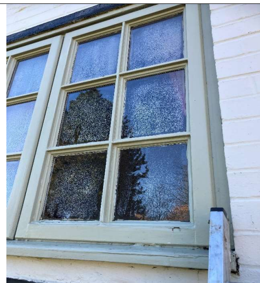
Window W3 showing projecting casements. Timber cill to be retained
