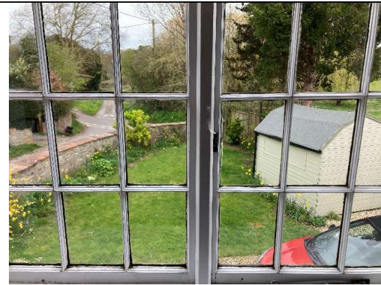
Window W1 internally
