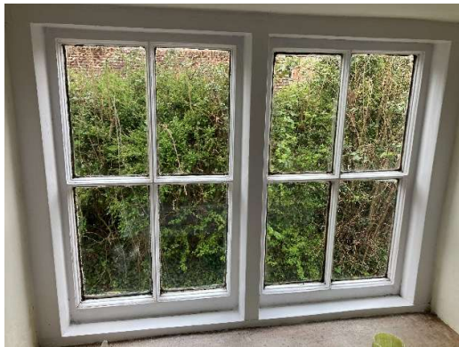
Window W4 internally
