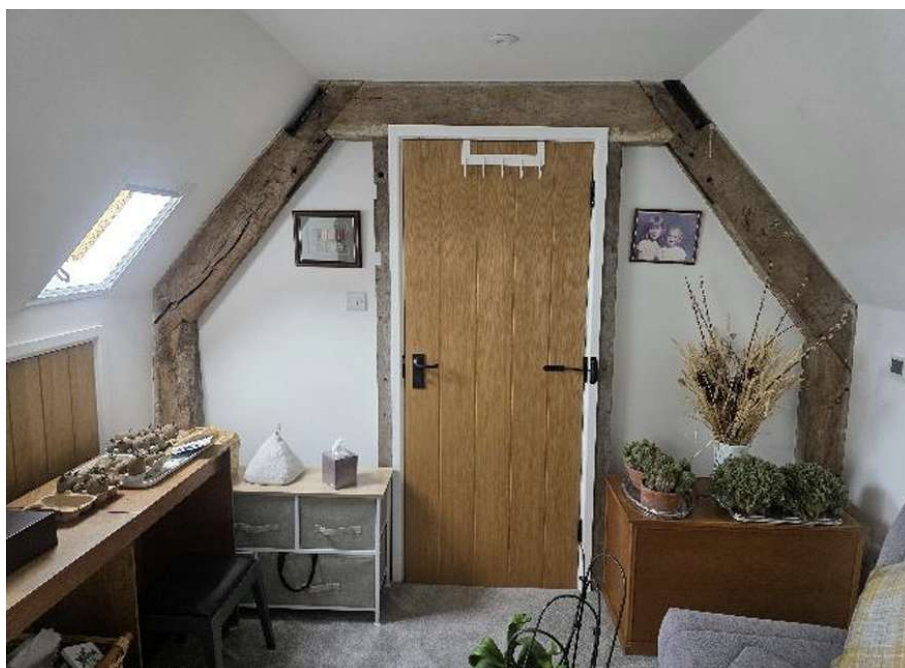
Figure 2 Bedroom in the roof space, facing north with the new partition between the bedroom and landing and staircase.
