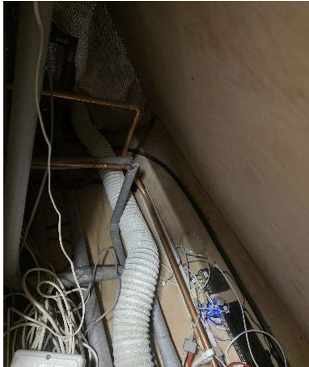
Figure 4 Services within the void at eaves level.
