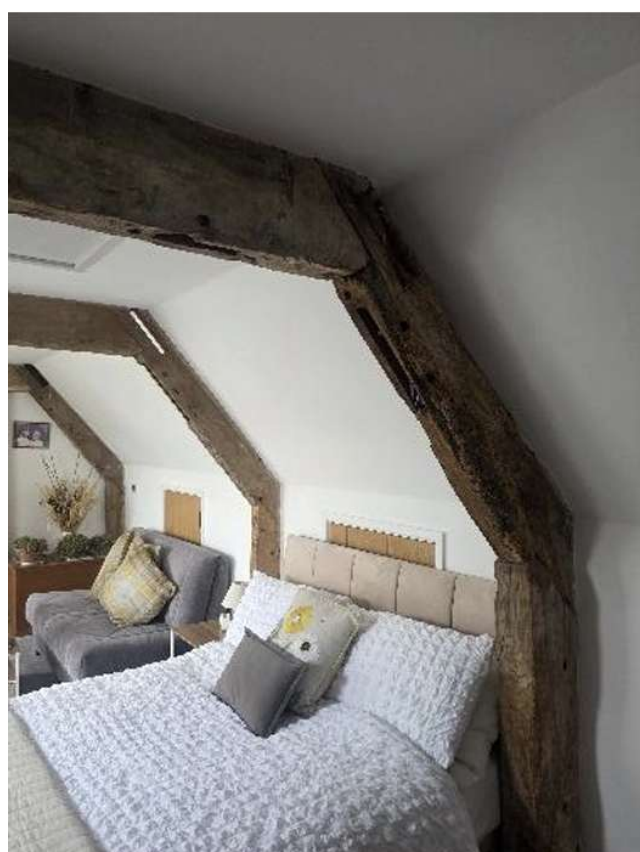
Figure 3 Detail of void mortices in the timbers of the roof.
