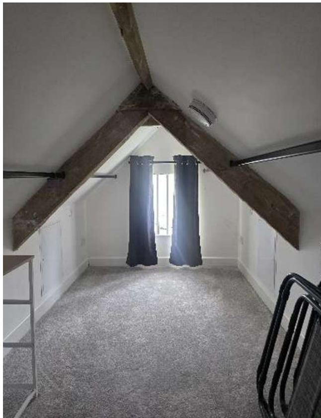
Figure 5 Attic space of the southern rear wing.
