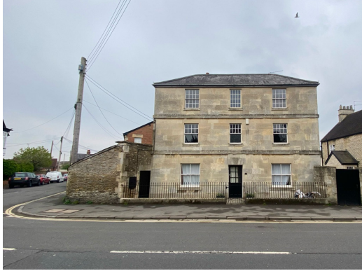
1. Looking West across Langley Road at the main elevation
