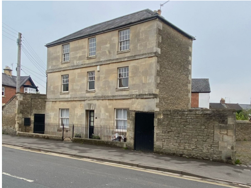
4. Looking north east along Langley Road
