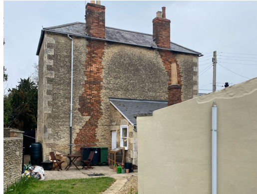
5. Rear blank elevation, with rear-most extension seen to right
