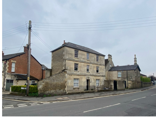
2. Looking south at the junction of Langley Road and Tugela Road
