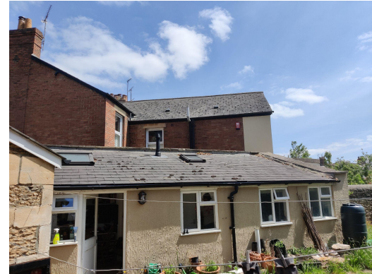
5. Side view of rear-most extension
