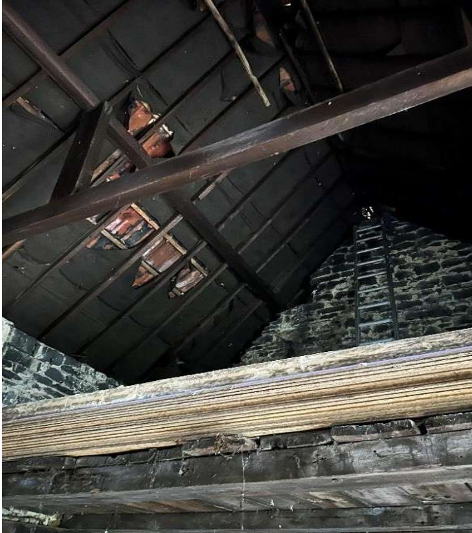
The internal roof void of the building.
