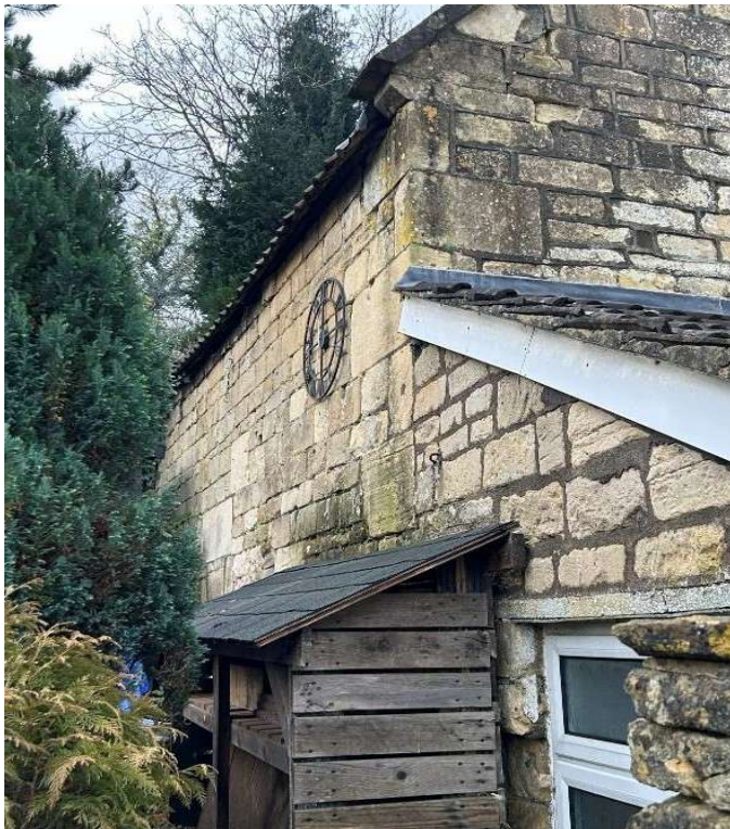
This photograph shows the rear of the building. And the integrity of the extension which is also devoid of soffits.
