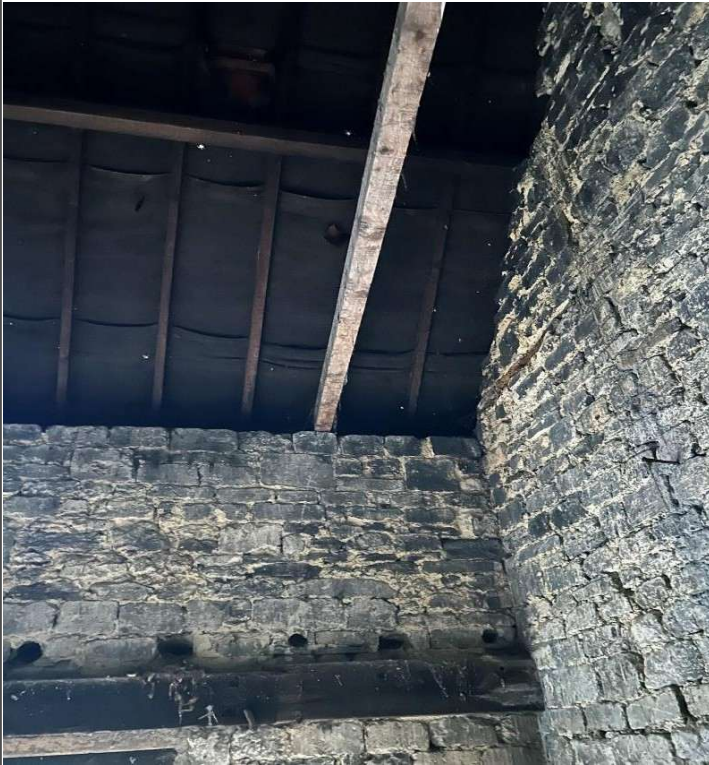
The internal roof void of the building.
