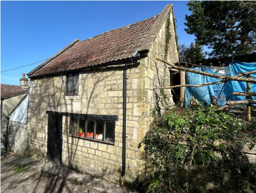
Side Elevation of Building
