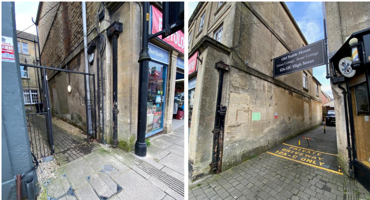
Site Visit – Existing gate between No's 14 and 16, and application site
