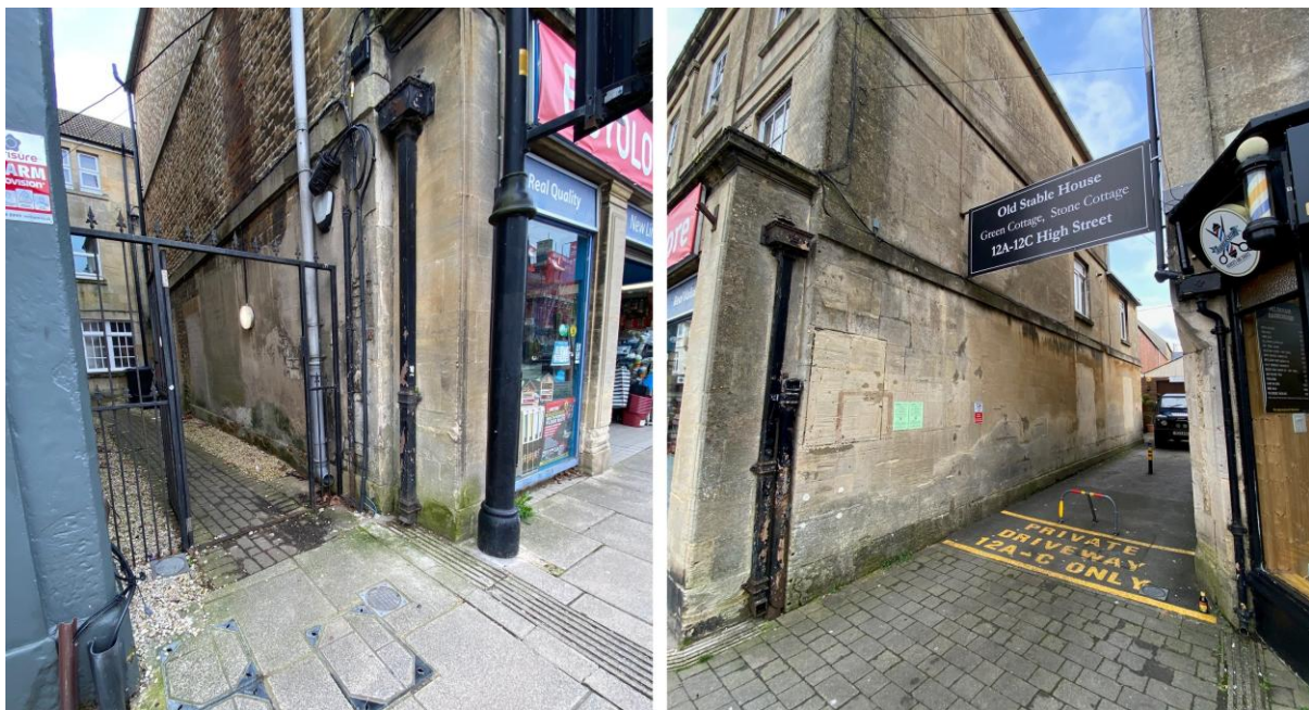
Site Visit – Existing gate between 14 and 16, and application site
