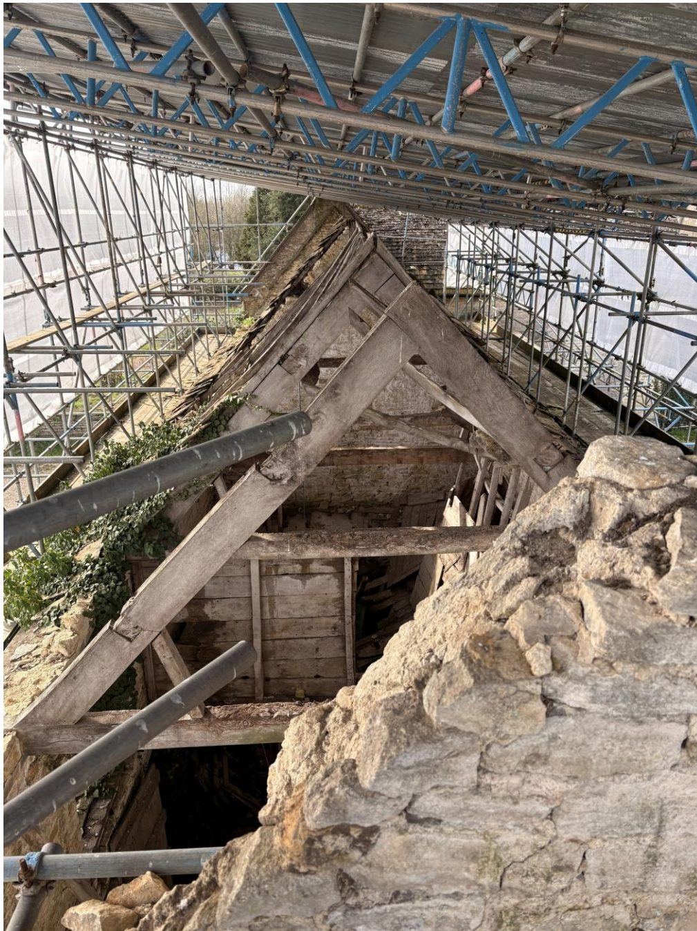
General View of Current Roof Structure – Photograph Taken From East Gable Looking West
