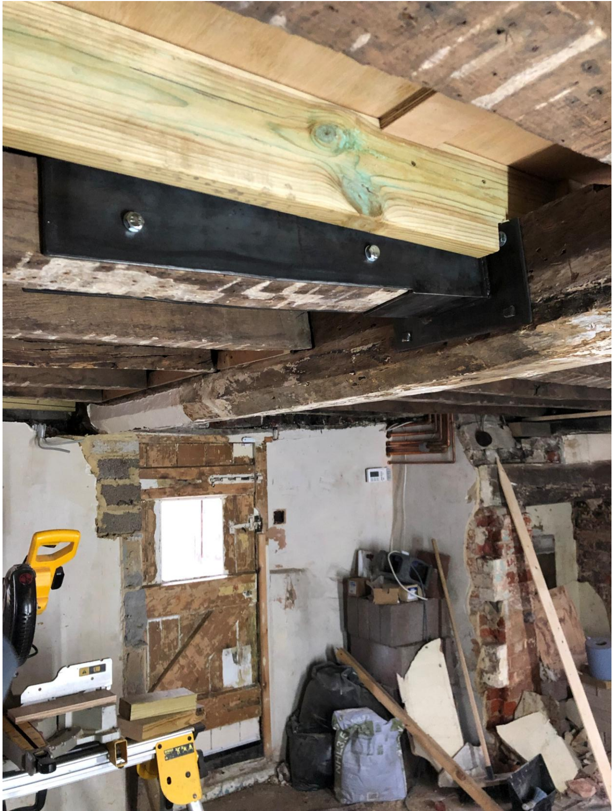
Possible Repair By Insertion of Local Bracketry
