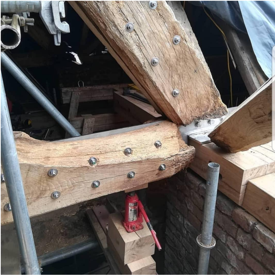
Possible Repair by Flitch Plate at Joints
