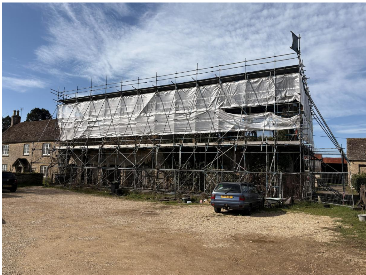
General Current View of Building Front Elevation
