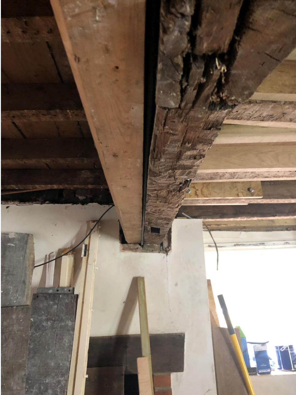
Possible Strengthening Of Beams By Steel Flitching
