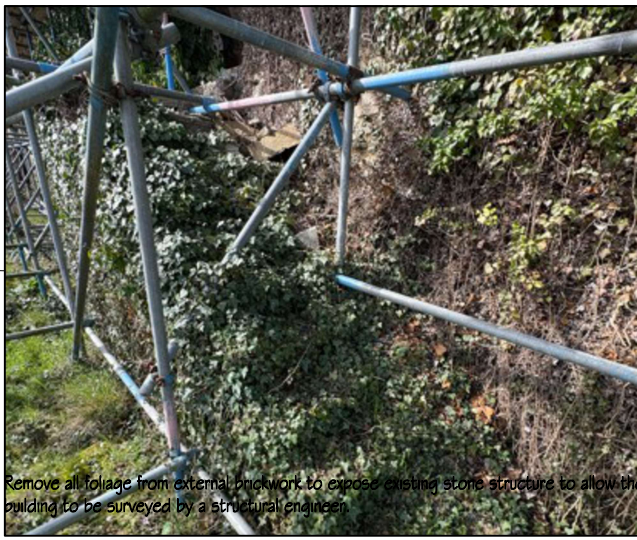
Remove all foliage from external stonework to expose existing stone structure to allow the building to be surveyed by a structural engineer.
