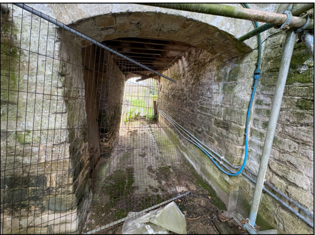
General view of passageway under listed building
