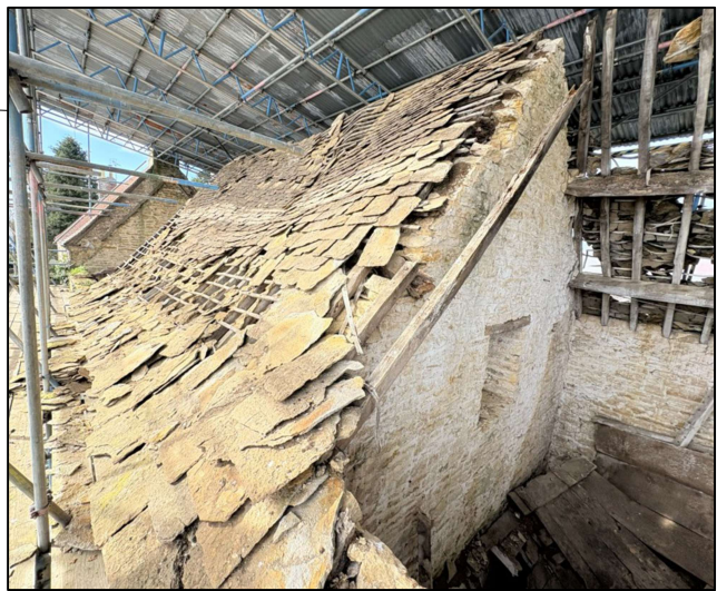
Section of existing roof with roof trusses and rafters in place.
