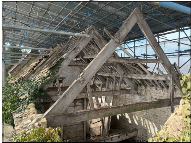
Section of existing roof with roof trusses and rafters in place.
