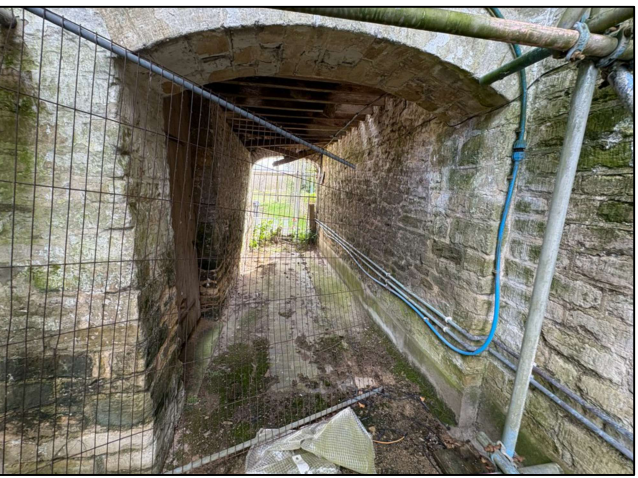
General view of passageway under listed building
