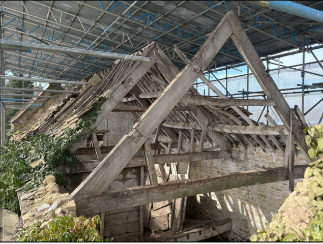
Section of existing roof with roof timbers and rafters in place.
