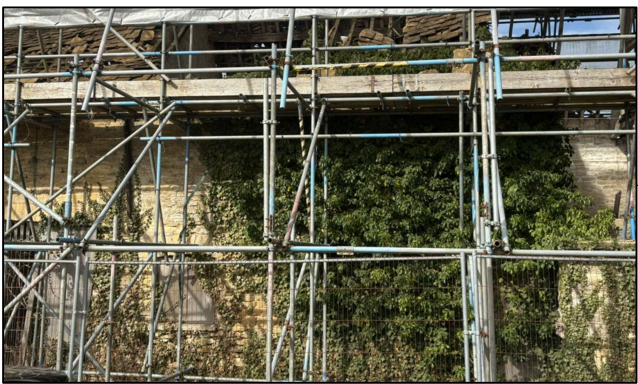
Remove all foliage from external brickwork to expose existing stone structure to allow the building to be surveyed by a structural engineer.
