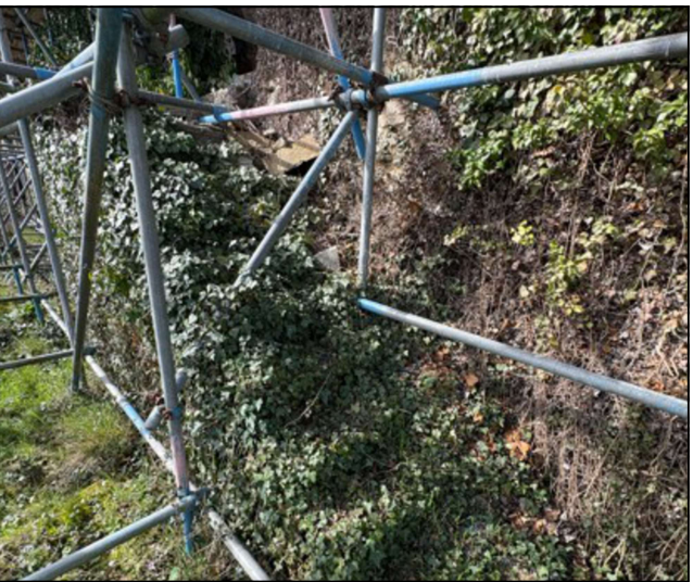
Remove all foliage from external stonework to expose existing structure to allow the building to be surveyed by a structural engineer.
