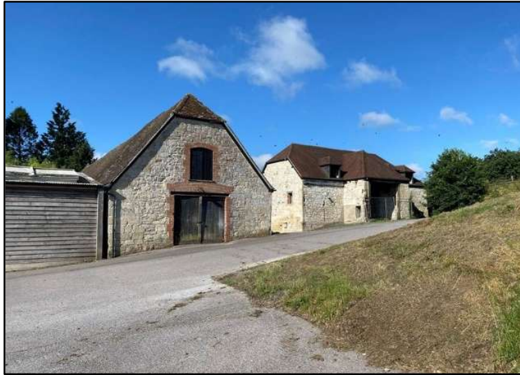
Figure 1: Right: Upper Kingstead Barn containing the cafe, tasting room and shop, Central: Listed Kingstead Barn (containing the distillery)
